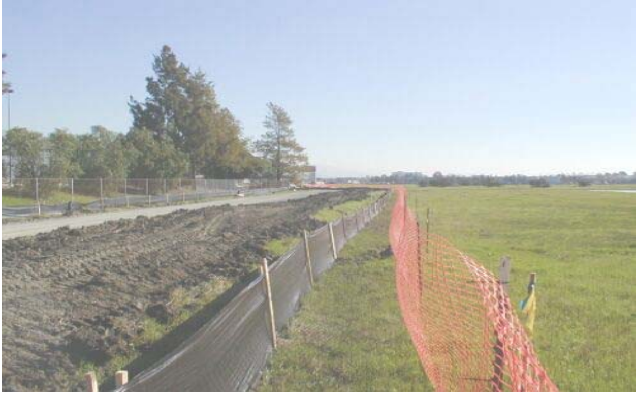
Figure 3 Staked Placed on Outside of Silt Fence for Access Road at Catella Property January 16, 2003
