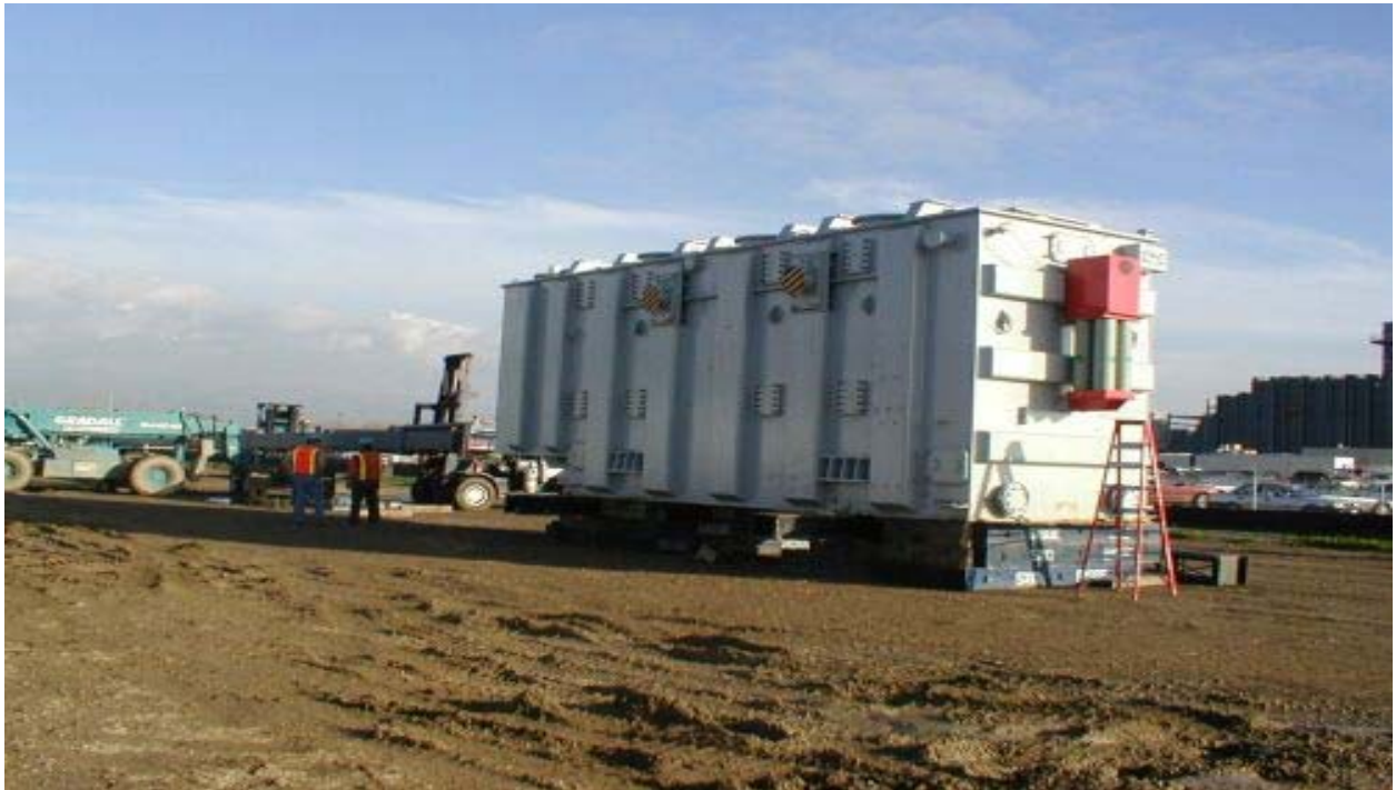
Figure 2 Arrival of Second Transformer at the Los Esteros Substation January 14, 2003
