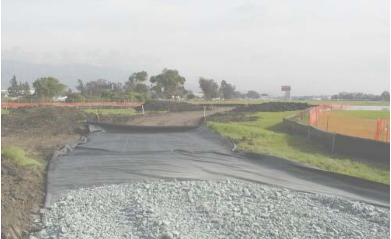
Figure 1 Access Road at Catella Property being Built for Foundation 5 January 14, 2003
