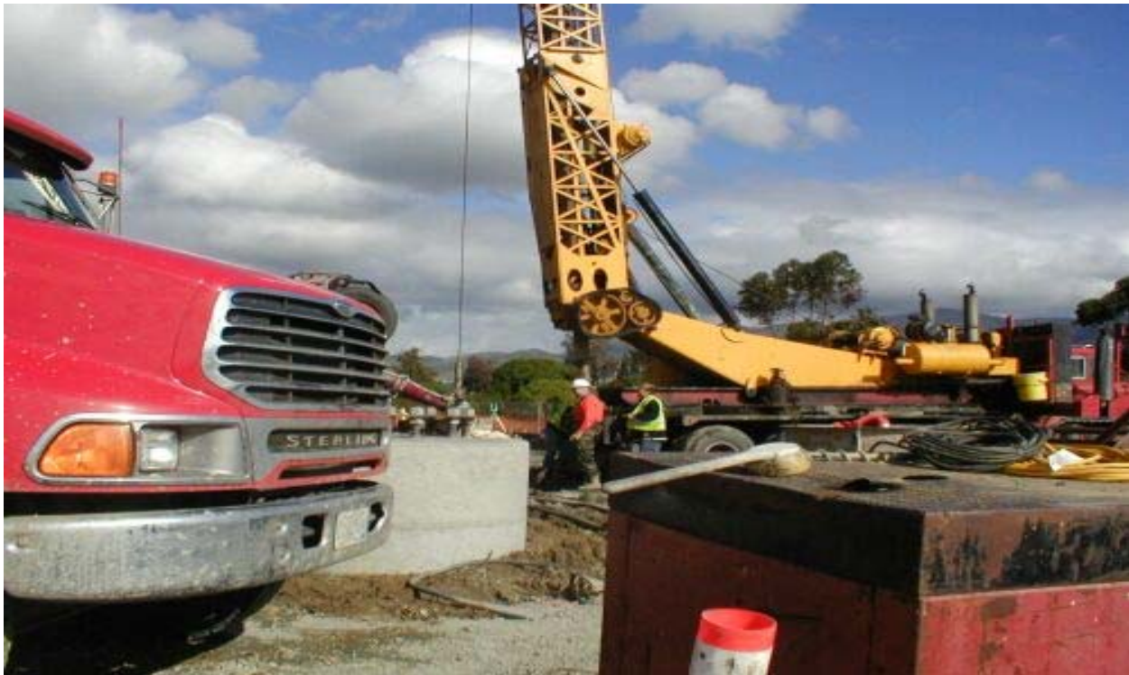
Figure 1 Pole Foundations 5 Being Built – Catella Property January 21, 2003
