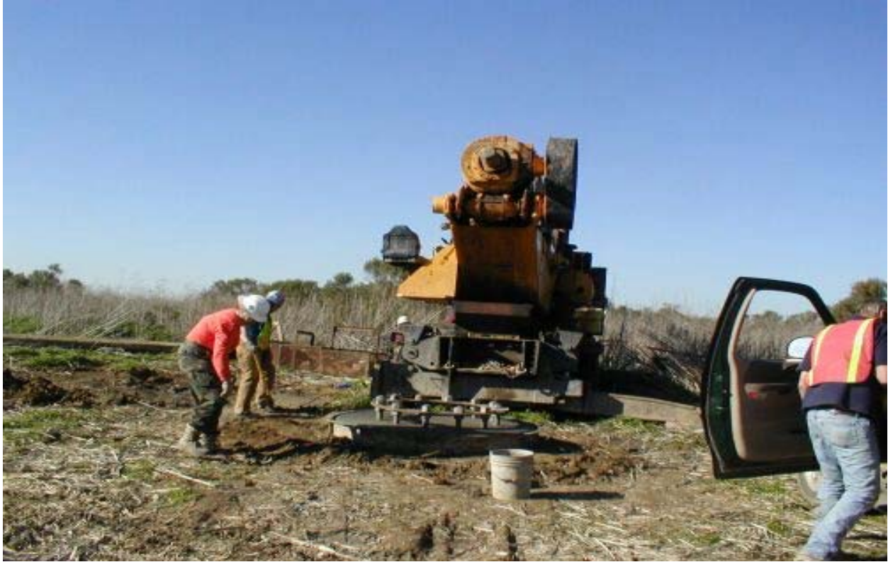
Figure 1 Tri-state Drilling – Pole Foundation #22 (WPCP) February 3, 2003
