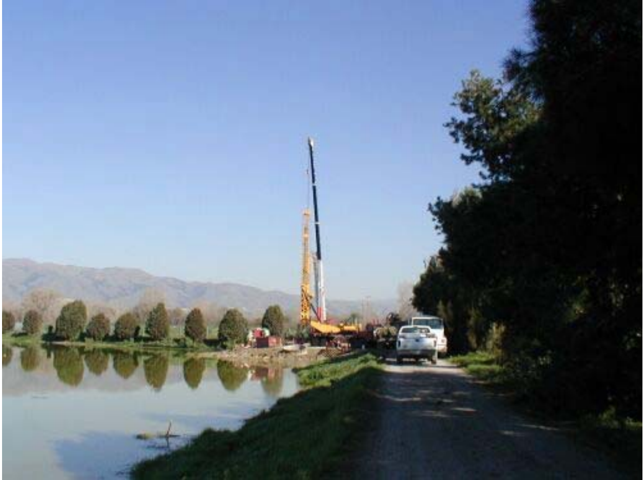
Figure 3 Tri-state Drilling - Pole Foundations #24(a) & (b) construction (WPCP) February 6, 2003
