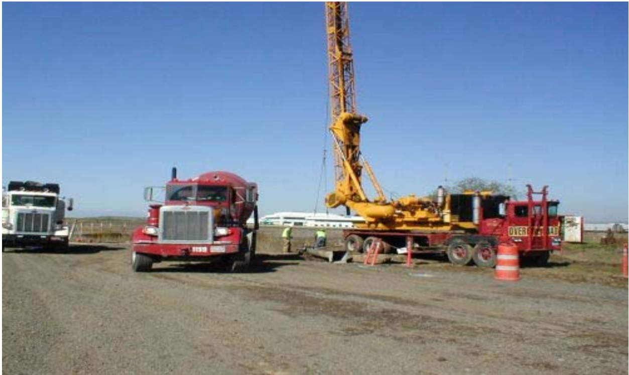
Figure 2 Tri-state Drilling at Pole area #11 on the King & Lyon's Property February 18, 2003
