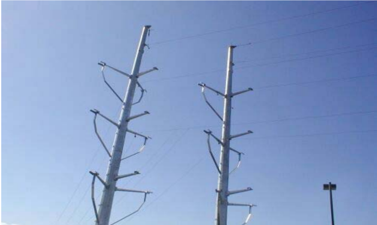
Figure 1 Poles #9(a) and (b) February 27, 2003
