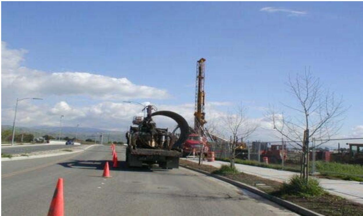
Figure 2 Tri-state Drilling at Pole area #14 along McCarthy Boulevard February 27, 2003
