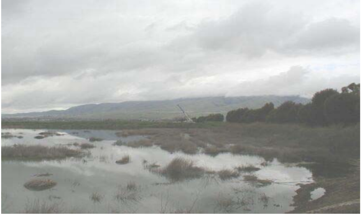
Figure 1 ILB Erecting Pole #20 at the WPCP – View Looking East, March 3, 2003
