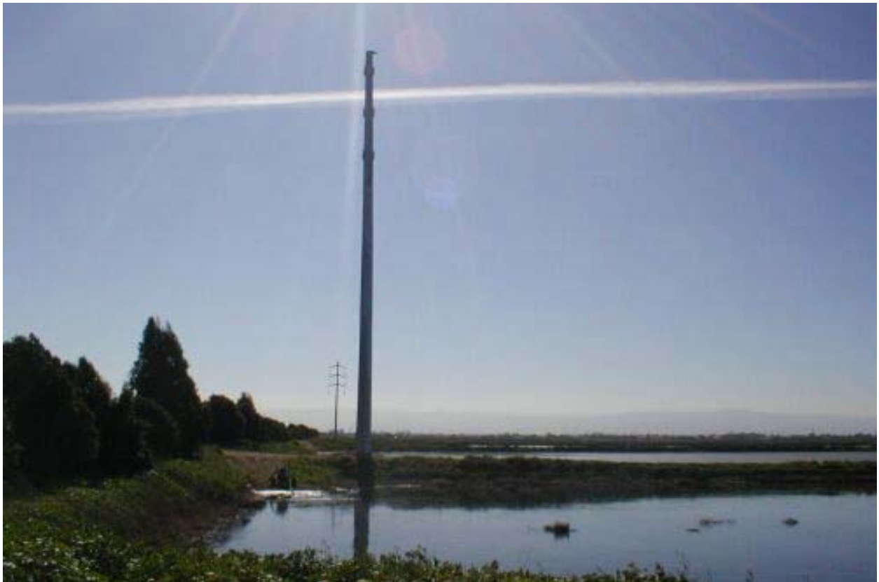
Figure 2 Poles at WPCP – View Looking West, March 6, 2003
