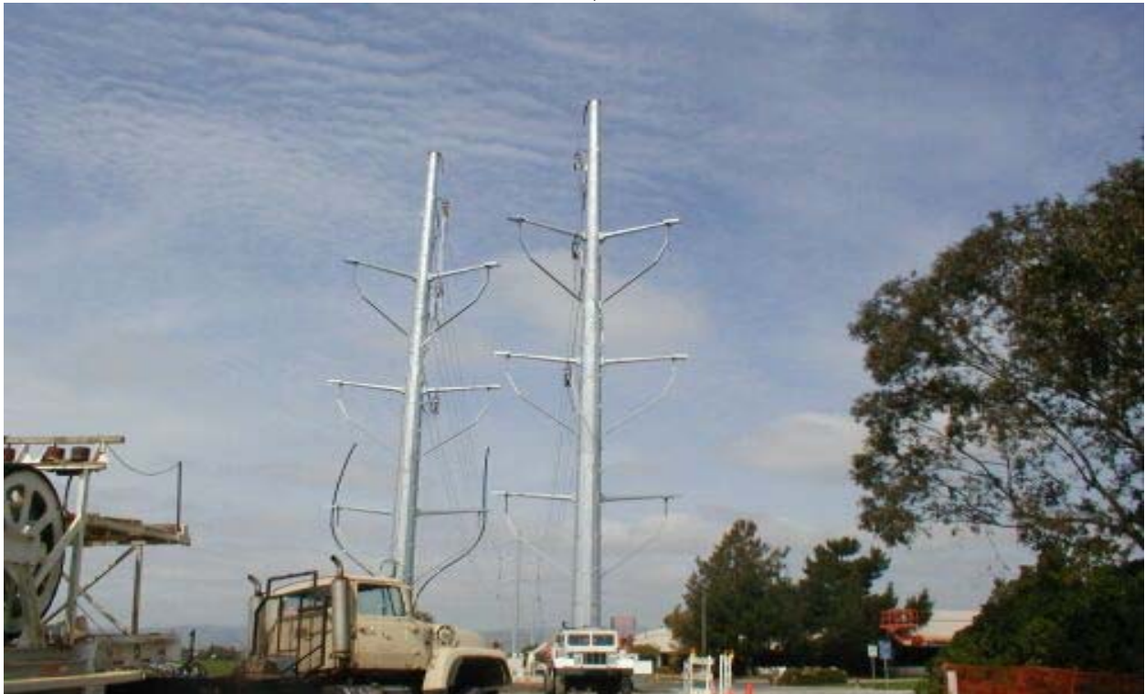
Figure 2 Poles #9(a) and (b) – Permanent Conductor Cable Pulled March 22, 2003
