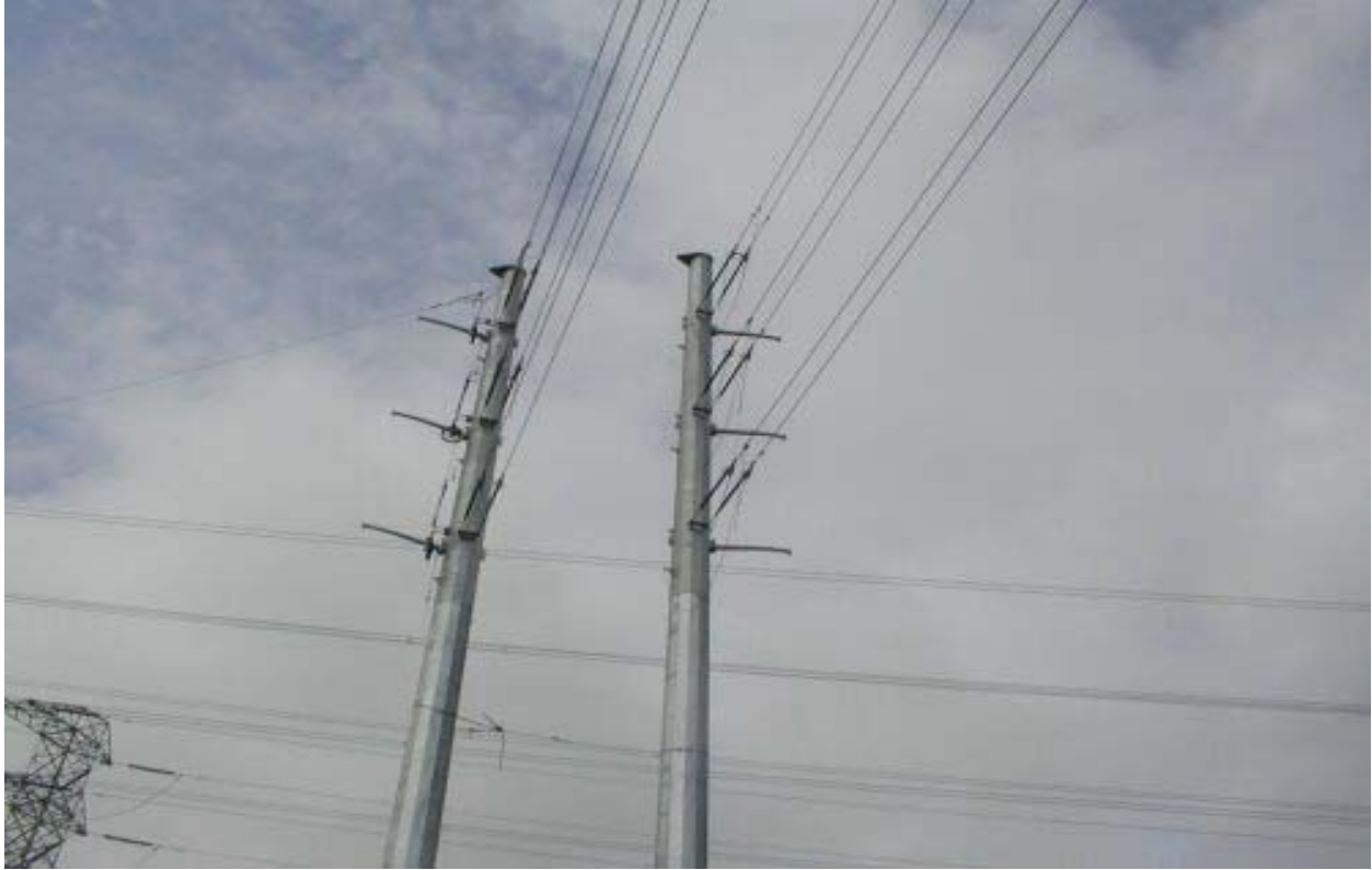
Figure 1 Poles #1 (a) and (b) – Permanent Conductor Cable Pulled March 22, 2003
