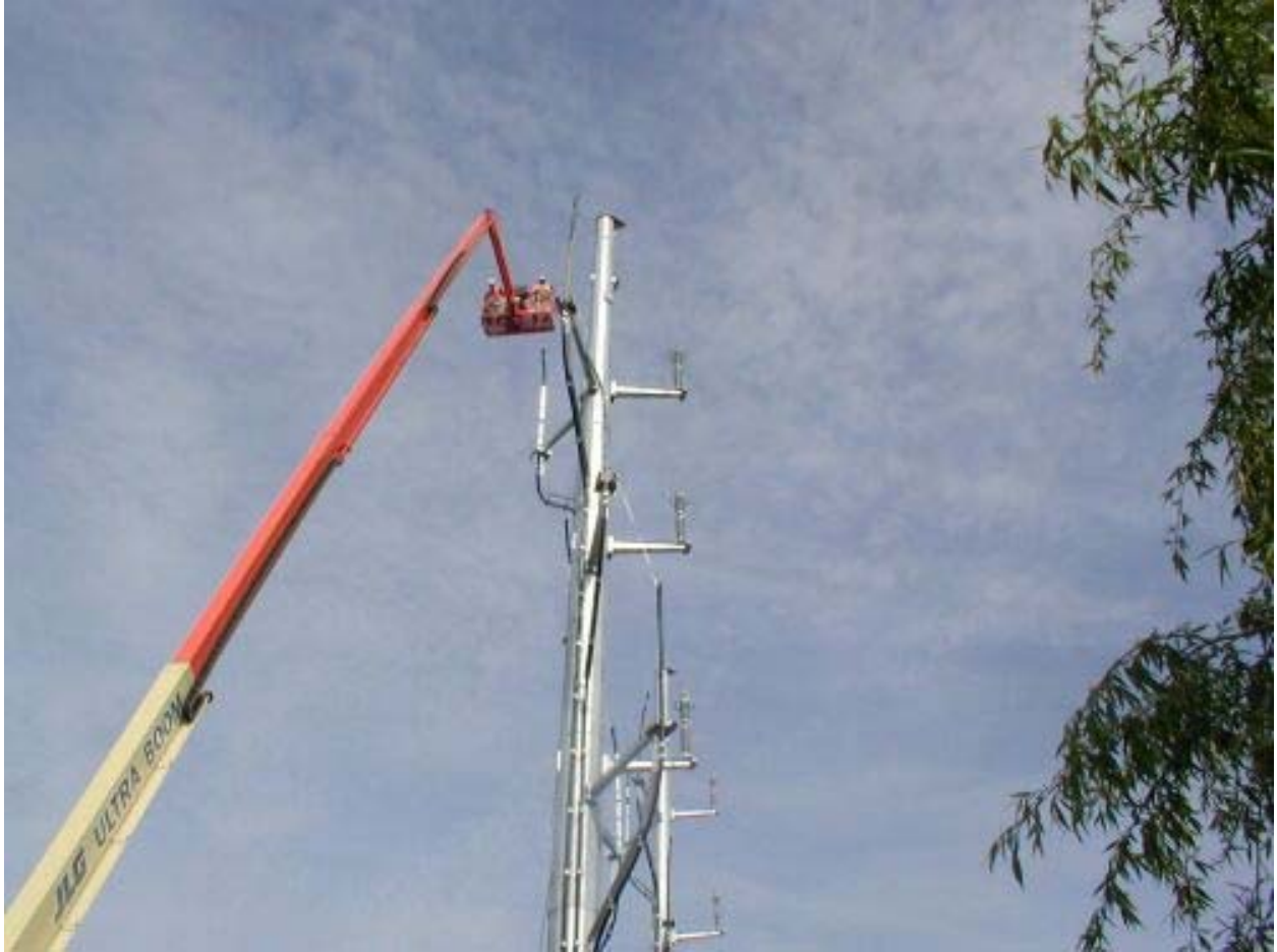
Figure 3 Crews Heating Cable at Pole #10 R March 22, 2003
