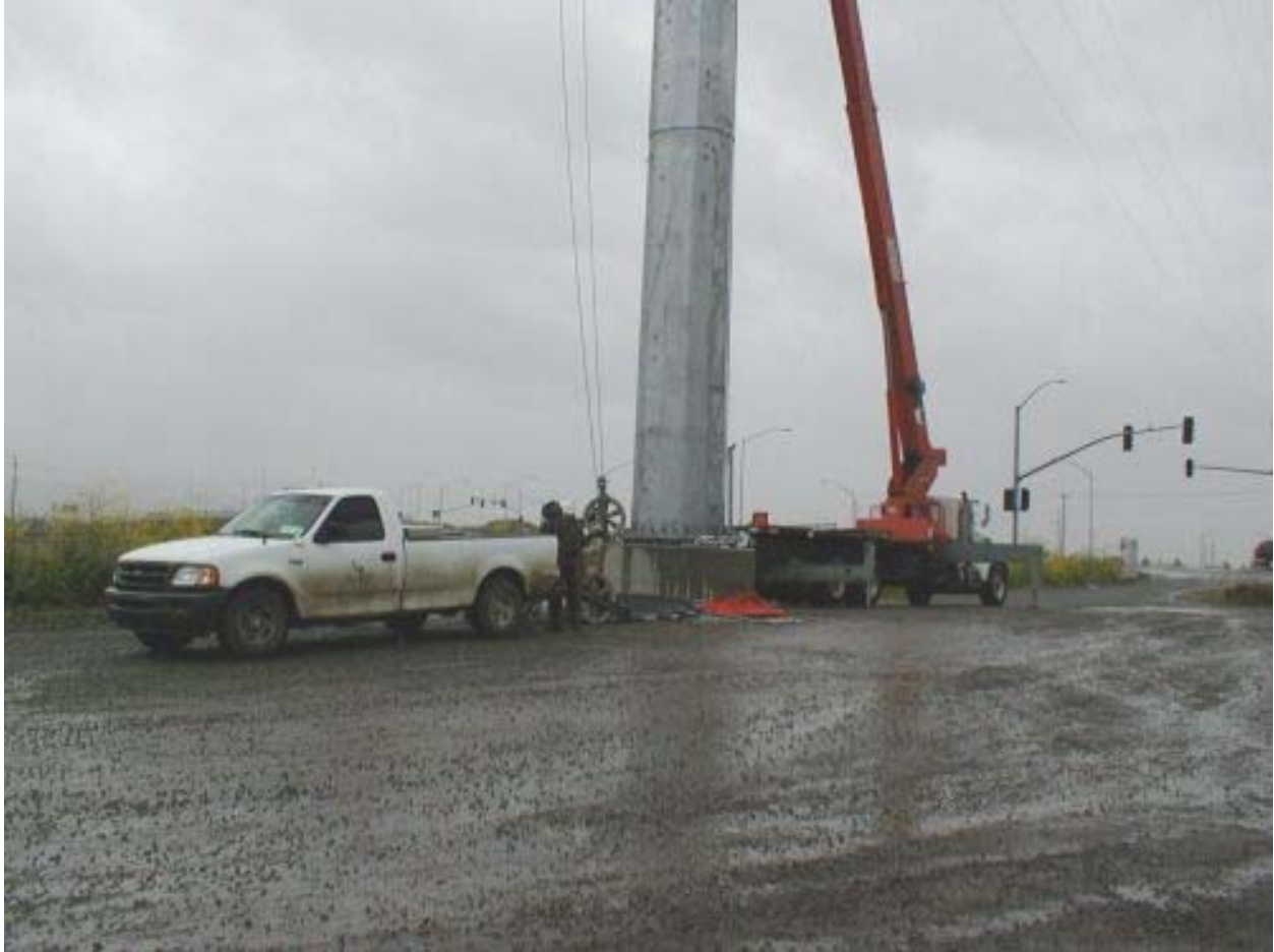
Figure 3 ILB Crews Working at Pole #13 on the King & Lyon's Property April 12, 2003
