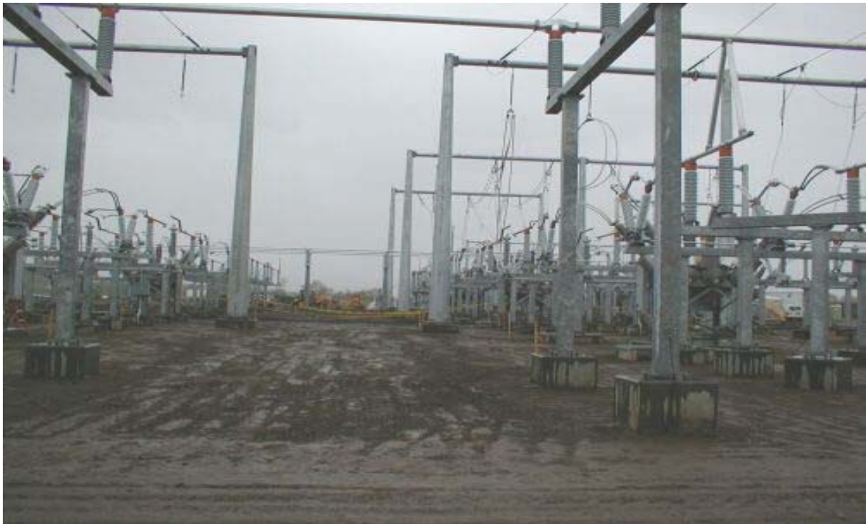
Figure 2 Los Esteros Substation Site April 12, 2003
