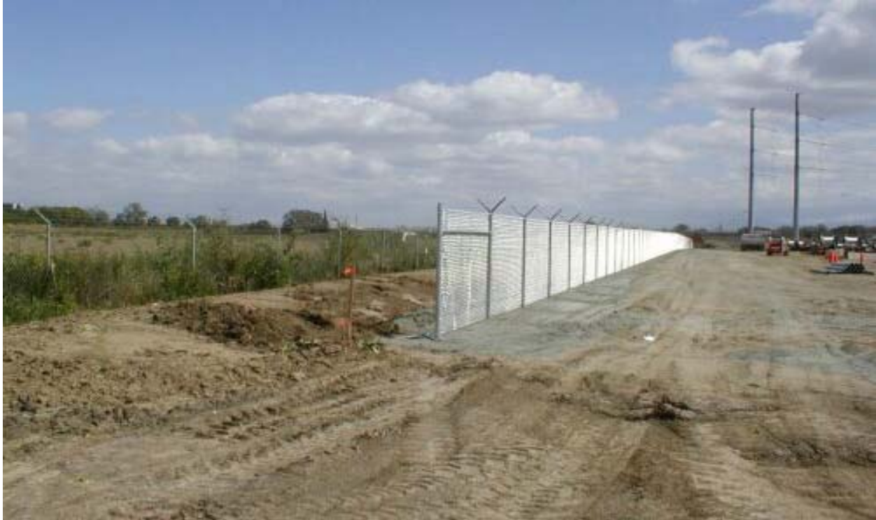
Figure 1 New Fence on East Side of the Los Esteros Substation May 7, 2003
