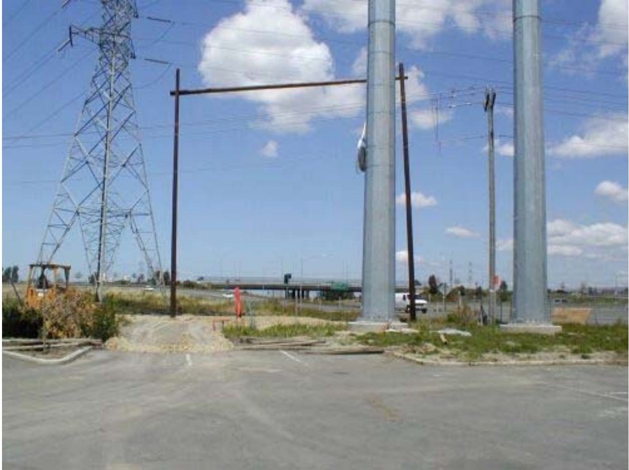
Figure 3 Crews Creating a Work Pad around Poles #1 L and R May 9, 2003
