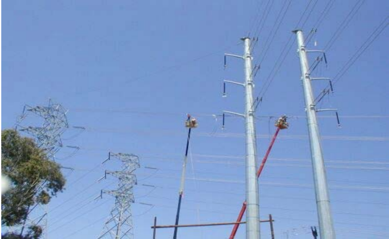
Figure 1 Crews Connecting Lines from Newark to NESJ May 12, 2003
