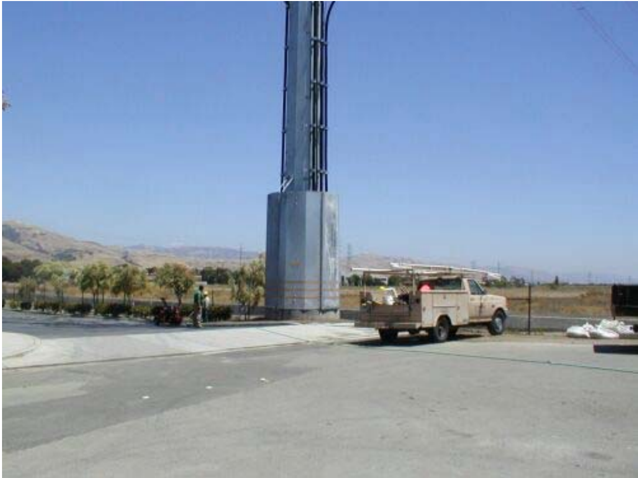
Figure 3 Landscaping Work at Poles #10 L and R June 20, 2003
