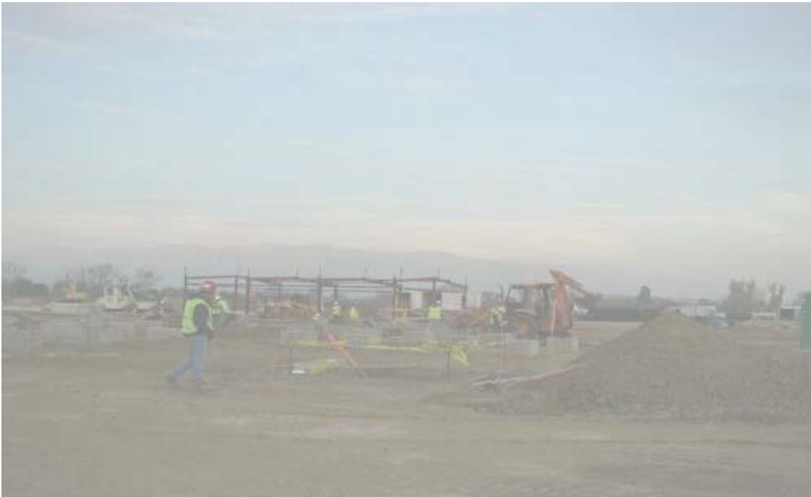
Figure 3 Los Esteros Substation: Operations Building Structure December 3, 2002
