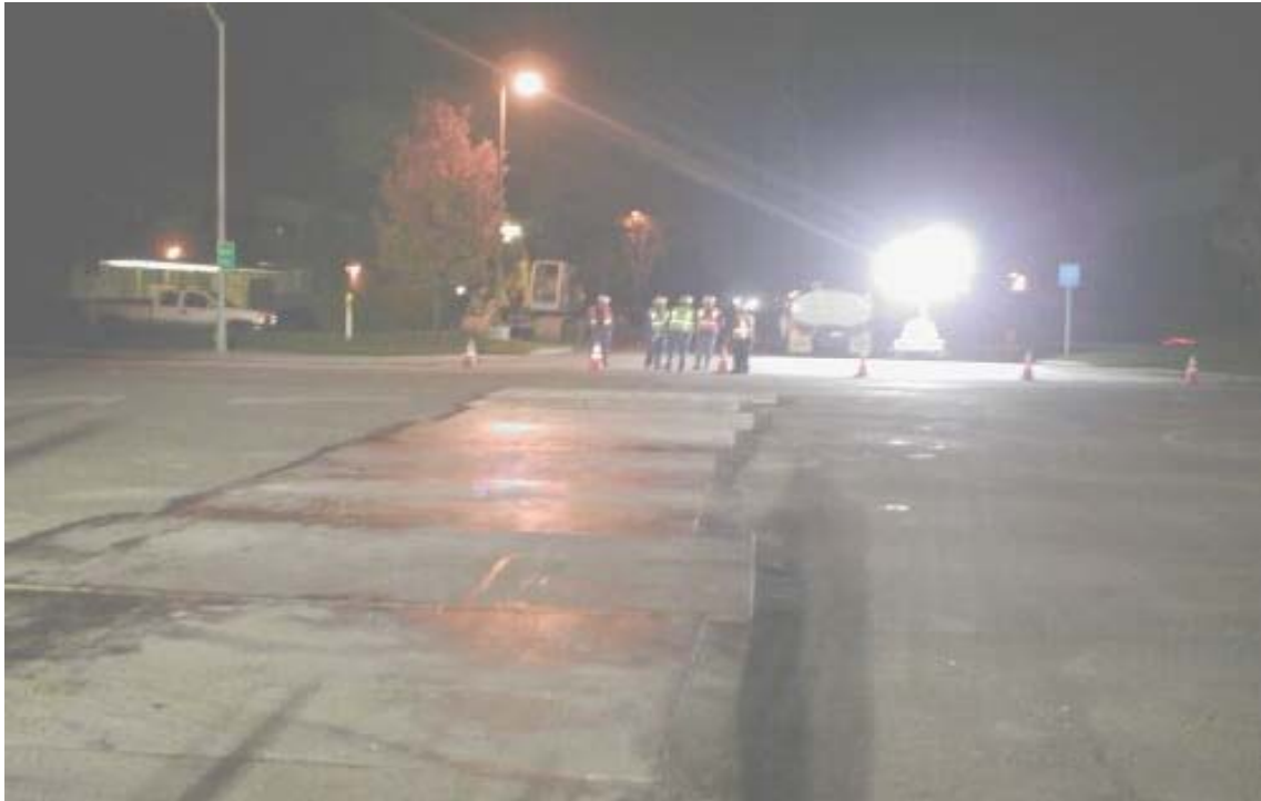
Figure 4 Crews setting up to trench across Gateway Boulevard. December 5, 2002
