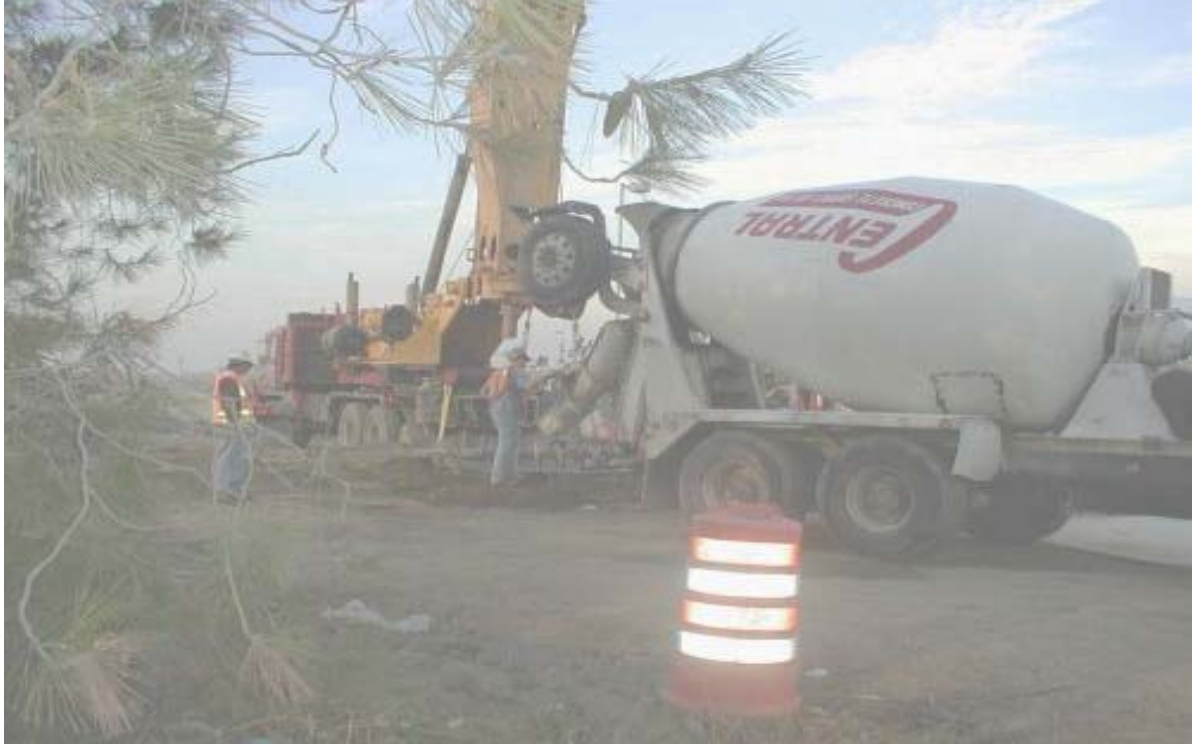
Figure 2 Pouring Foundation for Pole #16 December 3, 2002
