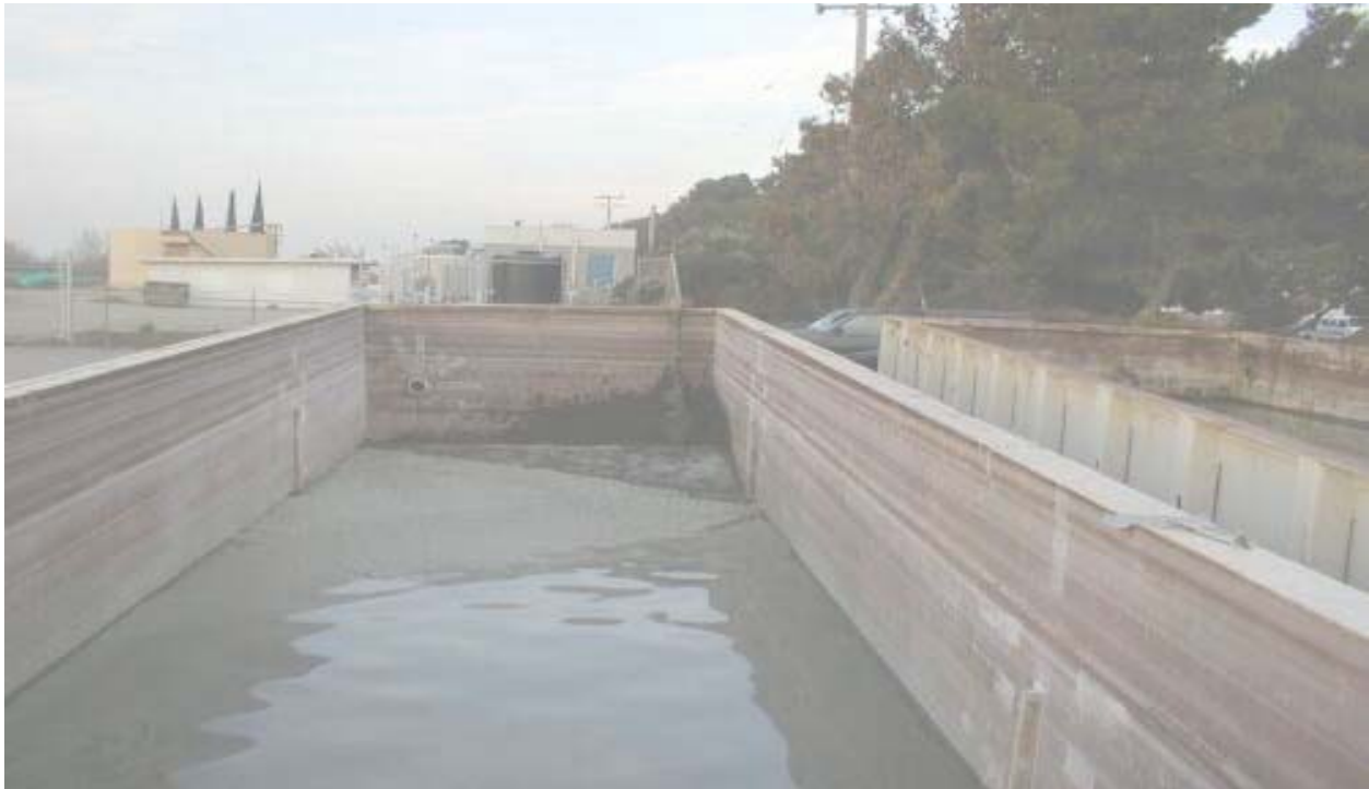
Figure 1 Baker Tanks at the Pole #17 Area December 3, 2002
