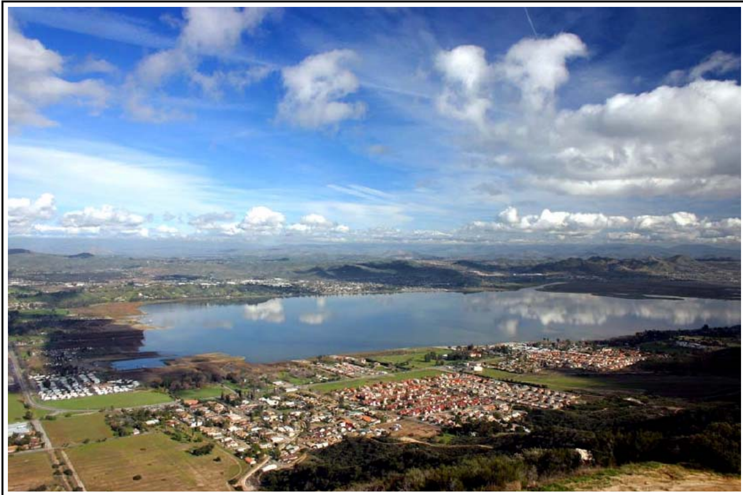
Figure 3-30 AERIAL PHOTOGRAPH OF EXISTING LOWER RESERVOIR (LAKE ELSINORE) Source: Elsinore Valley Municipal Water District
