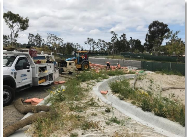
Figure 15. Curb and driveway restoration was conducted along Avenida Del Oro, May 7, 2019
