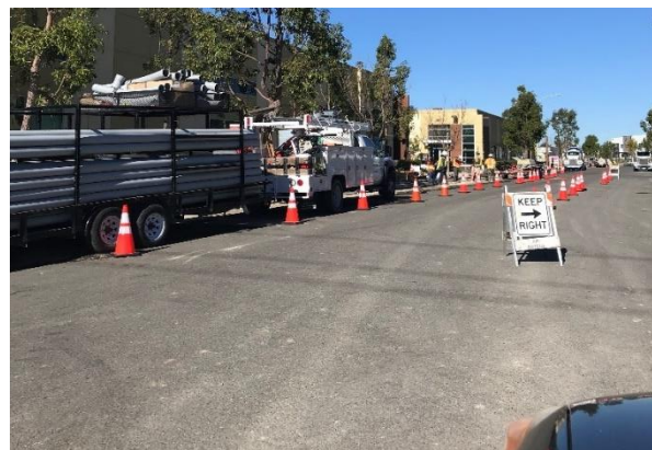
Figure 21. Traffic control set up for the 12 kV underground work along Rocky Point Drive, January 23, 2019
