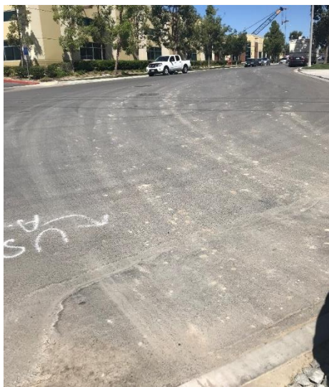
Figure 24. Trackout onto Rocky Point Drive from hauling activities, September 19, 2018
