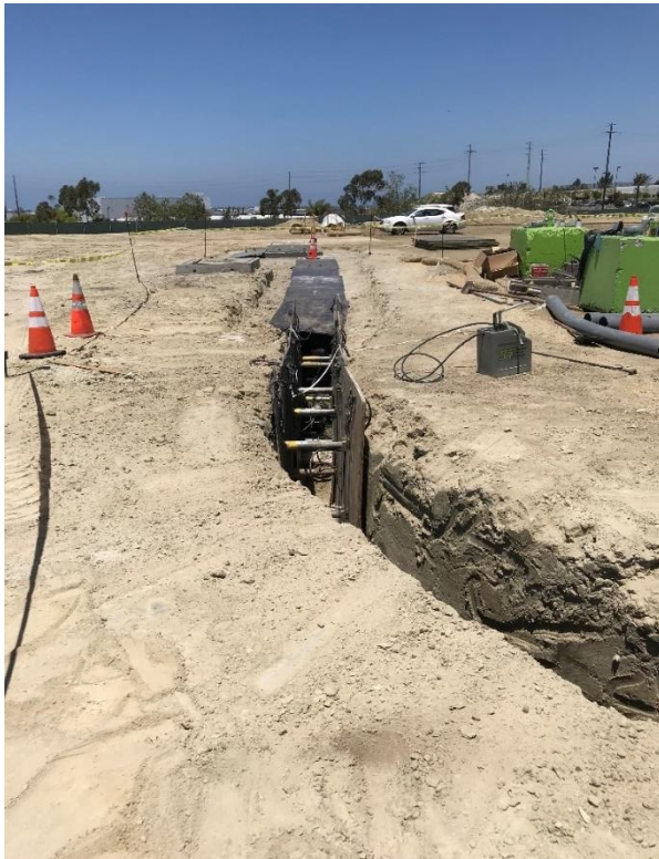
Figure 16. Trenching and conduit installation for the on-site distribution work continues
