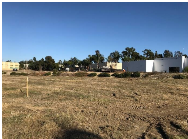
Figure 2. AM Ortega crews conducted vegetation mowing and tree removal at the Ocean Ranch Substation site
