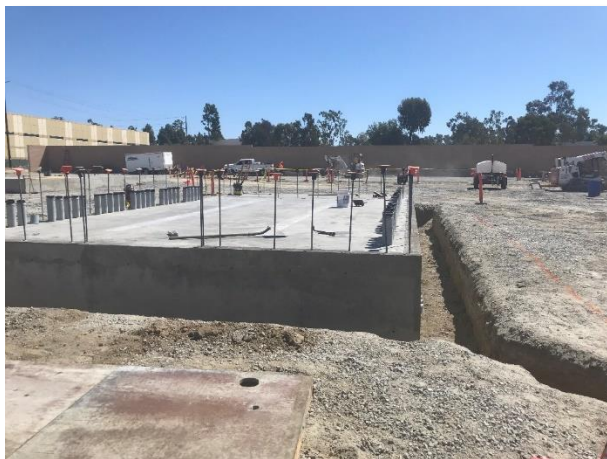
Figure 8. Concrete foundations built at the substation site, September 19, 2018
