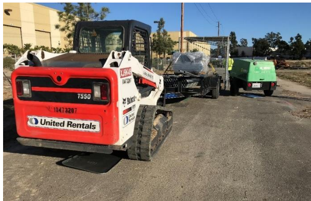
Figure 22. Equipment staged at the Ocean Ranch site with drip pans placed underneath
