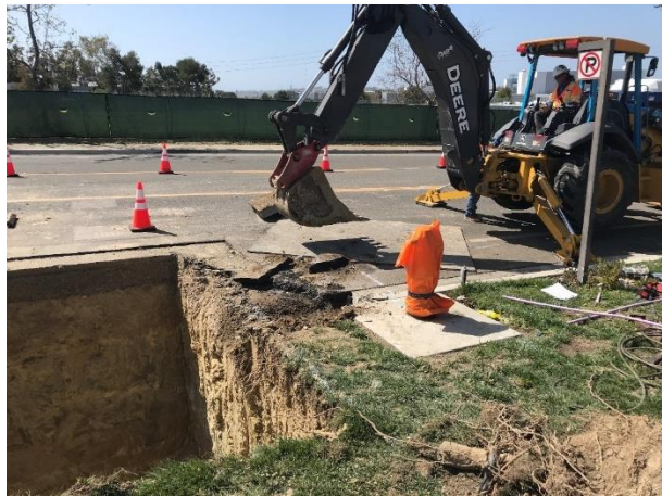
Figure 18. Vault excavation along Avenida Del Oro for the 12 kV work, March 13, 2019
