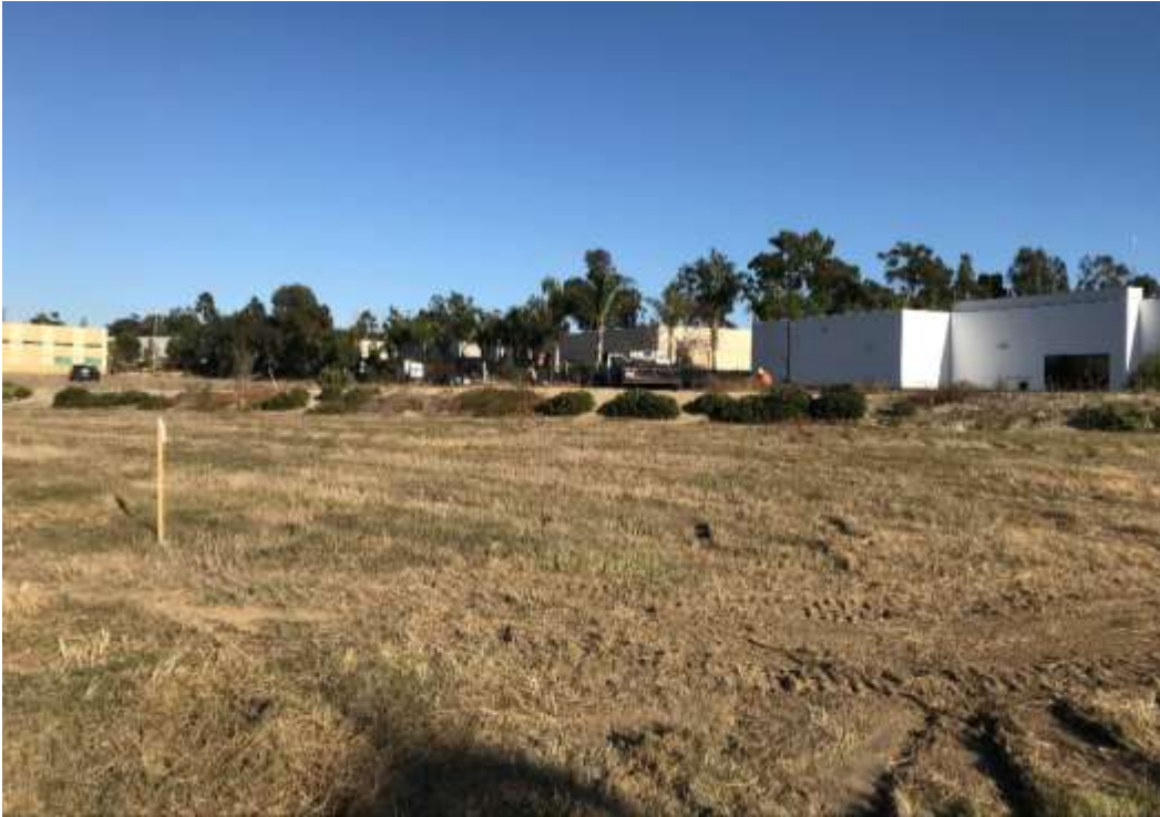
Figure 1 – AM Ortega crews conducted vegetation mowing and tree removal at the Ocean Ranch Substation site.
