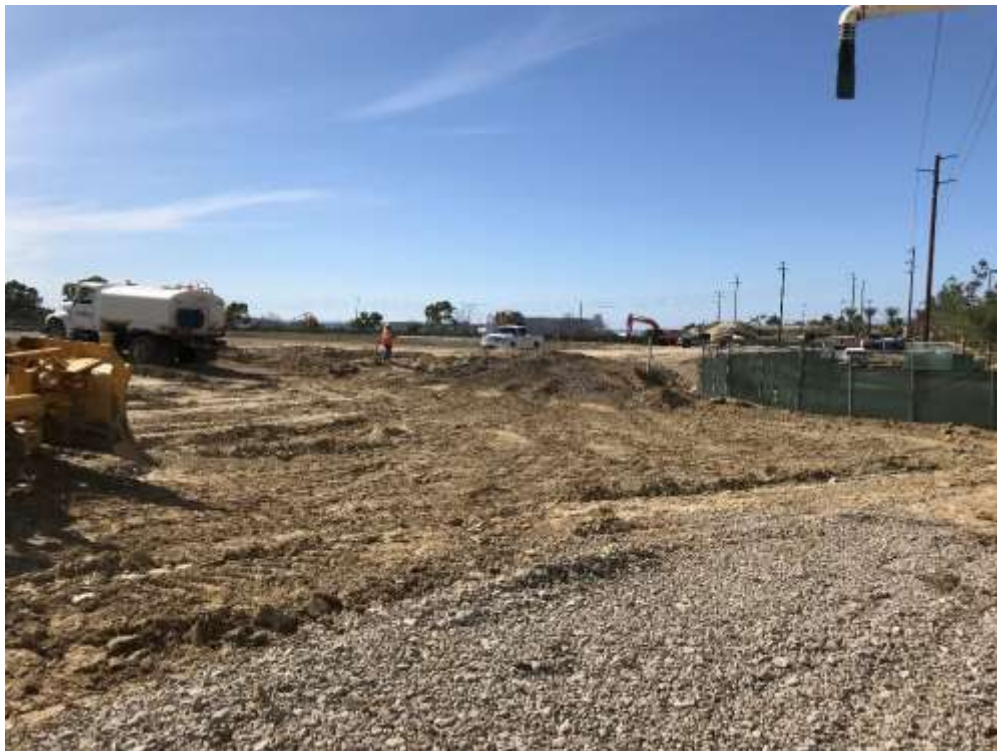
Figure 2 – Driveway preparation near the Substation entrance.
