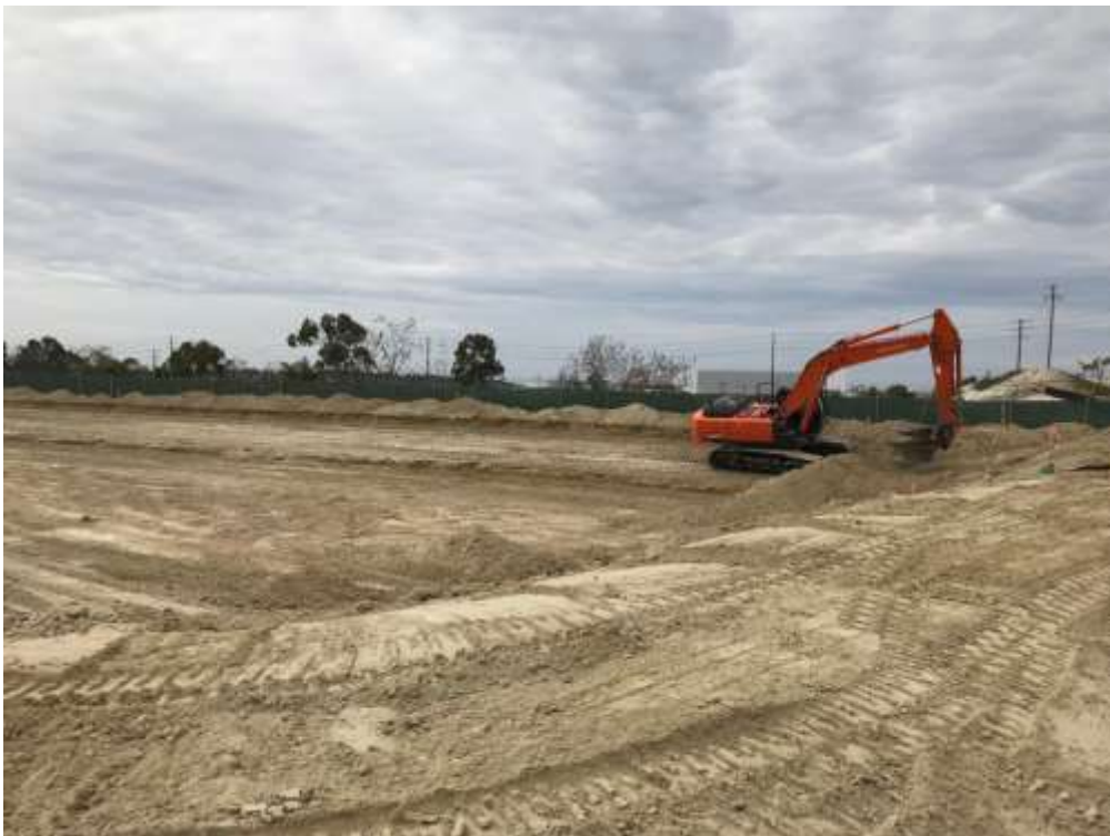
Figure 2 – Excavation of the large detention basin at the Substation site.
