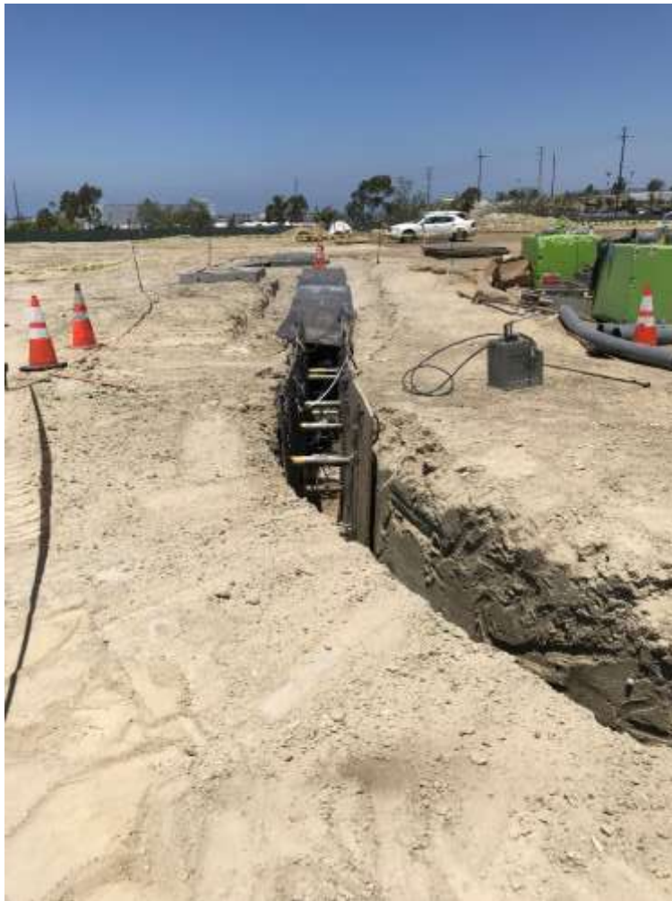
Figure 3 – Trenching and conduit installation for the on-site distribution work continues.
