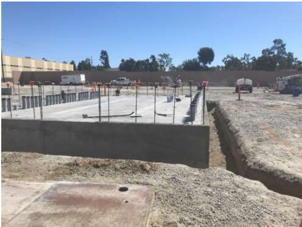
Figure 2 – Concrete foundations built at the substation site, September 19, 2018.
