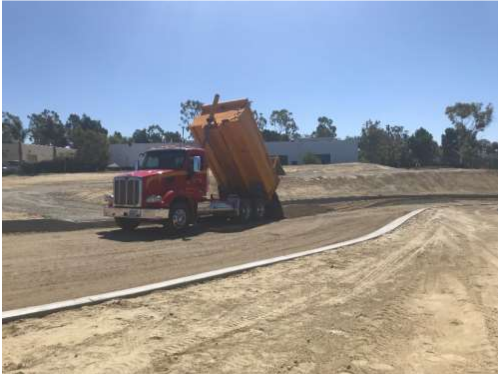
Figure 1 – Installation of base 2 rock along the substation driveway, September 19, 2018.
