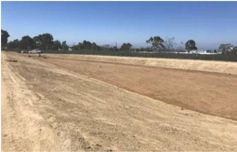
Figure 3 – Sediment controls, including straw wattles have been installed around the slopes of the detention basins, September 19, 2018.
