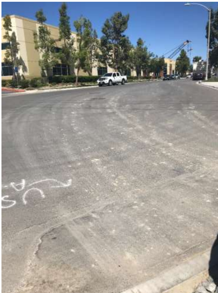
Figure 4 – Trackout onto Rocky Point Drive from hauling activities, September 19, 2018
