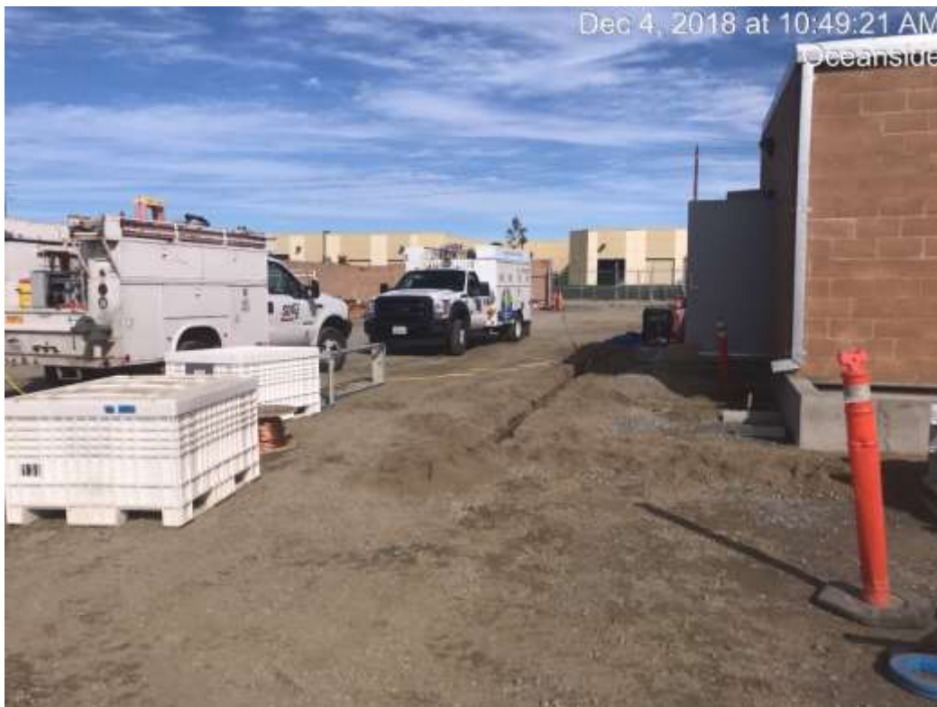
Figure 2 – Trenching of underground substation components occurred during the subject period, December 4, 2018.
