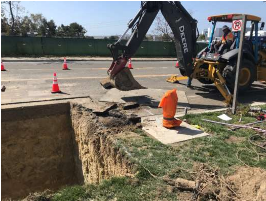
Figure 3 – Vault excavation along Avenida Del Oro for the 12-kV work, March 13, 2019.
