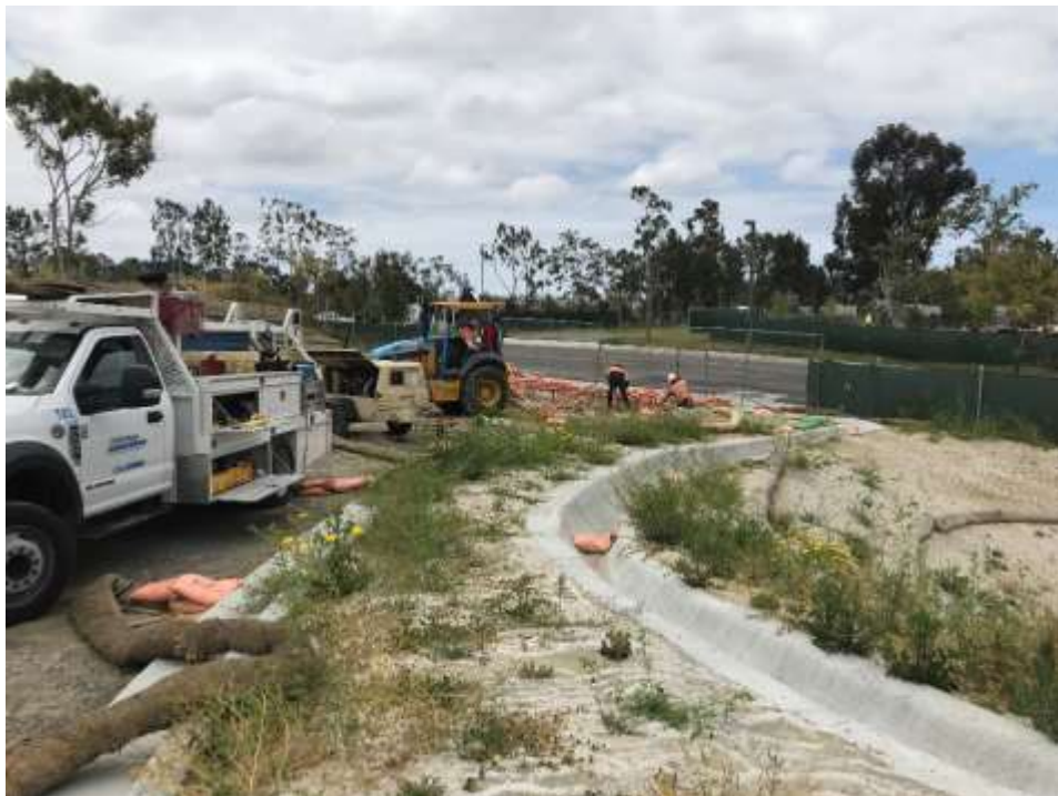
Figure 2 – Curb and driveway restoration was conducted along Avenida Del Oro, May 7, 2019.
