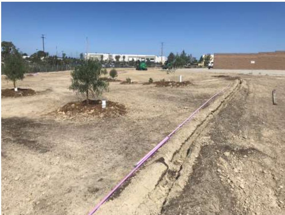
Figure 2 – Lateral irrigation line installation surrounding the low-profile Ocean Ranch Substation, October 4, 2019.
