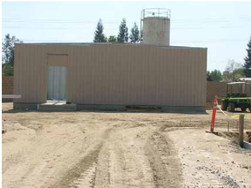
Figure 2: The Mechanical Electrical Equipment Room (MEER), which will be the only permanent building on site, was in place, and will be equipped during the electrical construction phase of the Project. The photograph faces southward.
