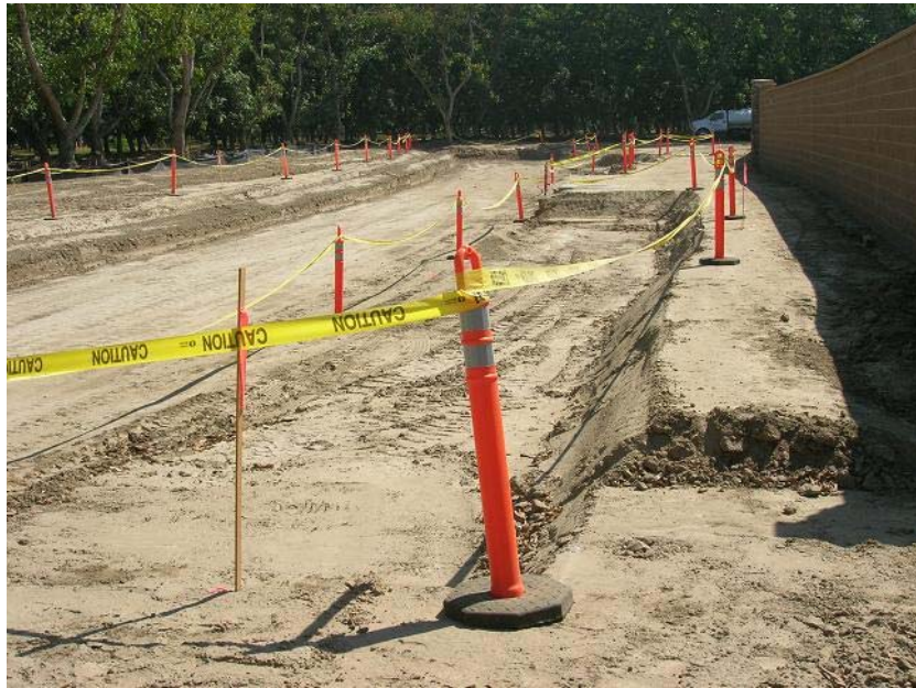
Figure 3: Some work was done on the retention basins prior to the current work stoppage. The road under construction is on the left; one of the retention basins is in the middle; the perimeter wall of the station is on the right. The photograph faces eastward.
