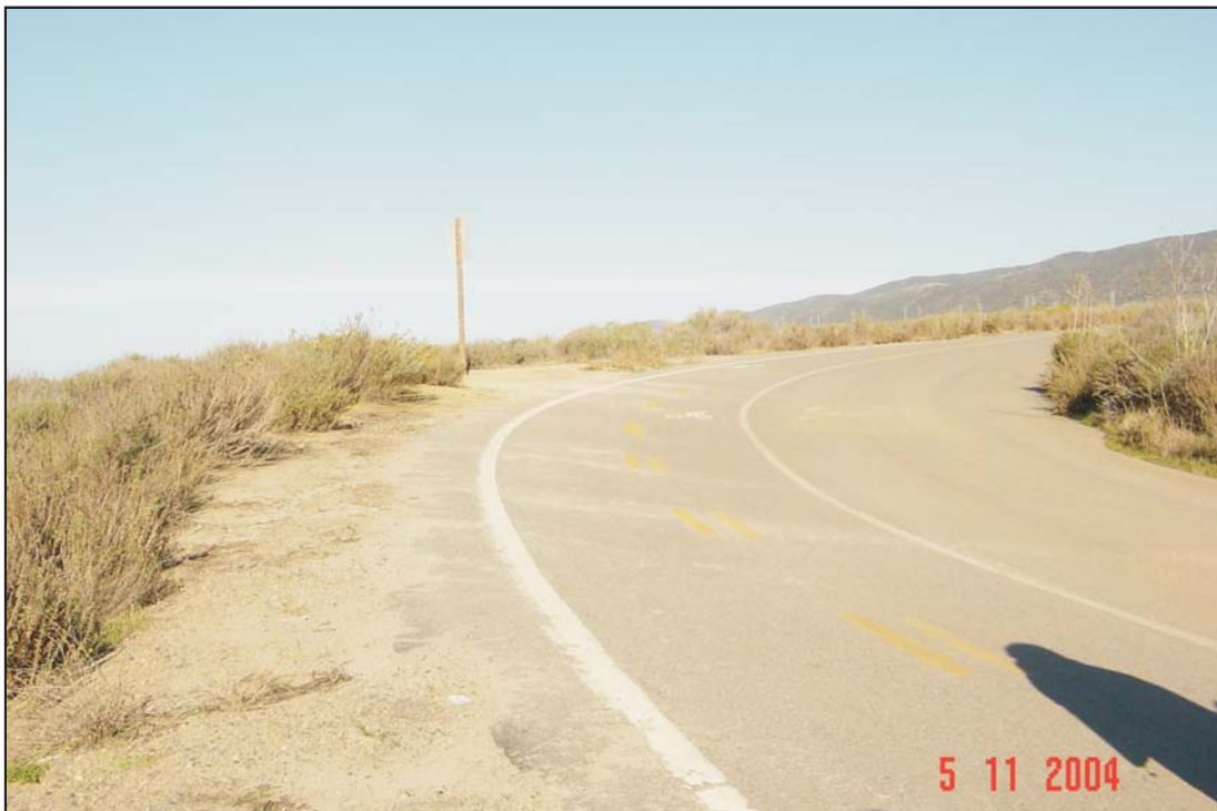
Looking northeast on Old Highway 101 at the "Y" turn.
