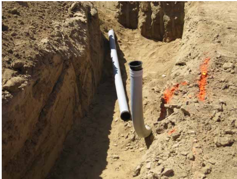
Figure 5: One partially buried pipe with a diameter of six inches (similar to, but with larger diameter than the one photographed) was left open over night accidentally. A plug was gently pushed through the pipe to the other open end, under supervision by the biological monitor, to ensure no animal was present. The pipe then was closed.
