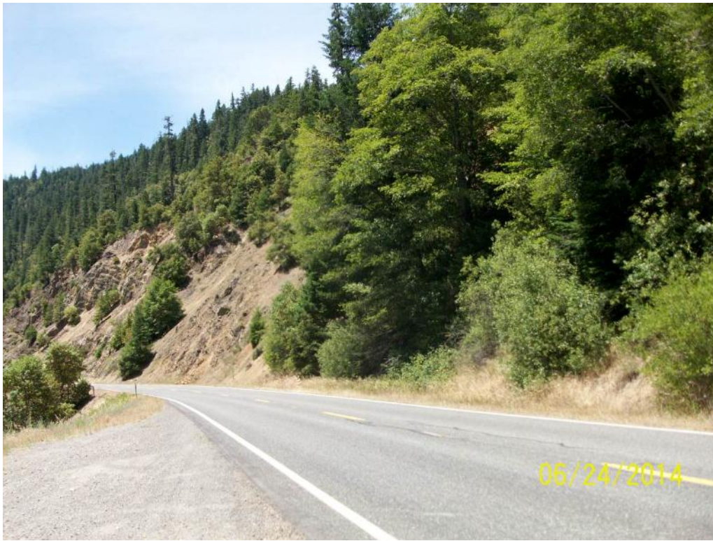
Photograph 1. Typical ROW habitat at approximately MP 28.00. No special-status plants were observed.
