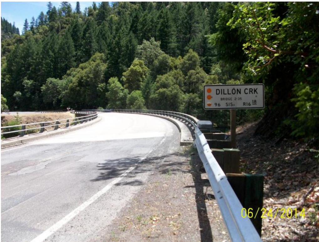
Photograph 4. Dillon Creek Bridge. Cables would be attached to the bottom of the structure to avoid disturbance to the creek.
