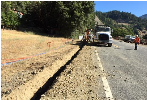
Figure 4. Crew trenching in conduit at MP 28.5 (July 24, 2019)
