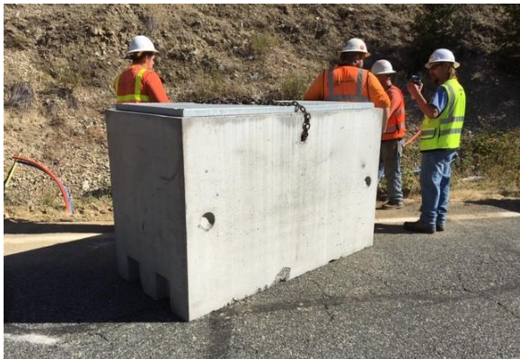
Figure 2. Crew installing tie-in box at MP 24.08 (July 10, 2019)
