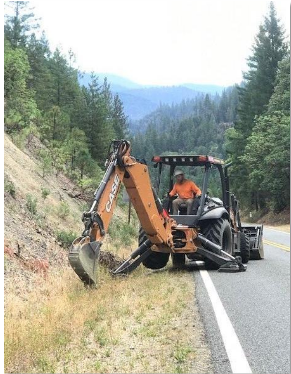
Figure 7. Crew excavating a pit to clean up a frac-out at MP 29.8 (August 28, 2019)
