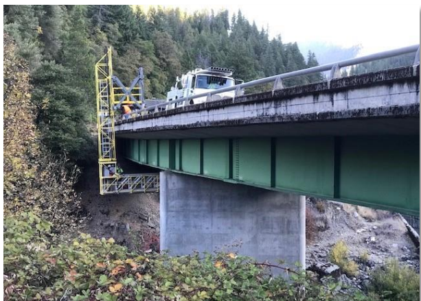
Figure 5. Bridge handling operations at Clear Creek Bridge (October 9, 2019)
