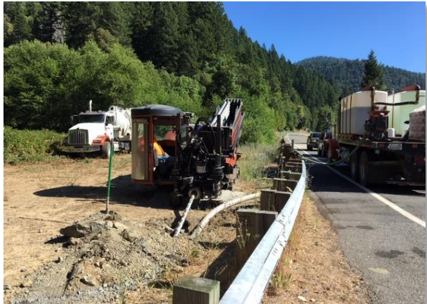
Figure 3. Crew boring south of Swillup Creek at MP 23.25 (July 24, 2019)
