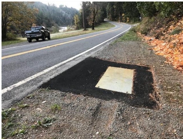
Figure 11. Clean drill and tie-in location in Phase 1 (October 31, 2019)
