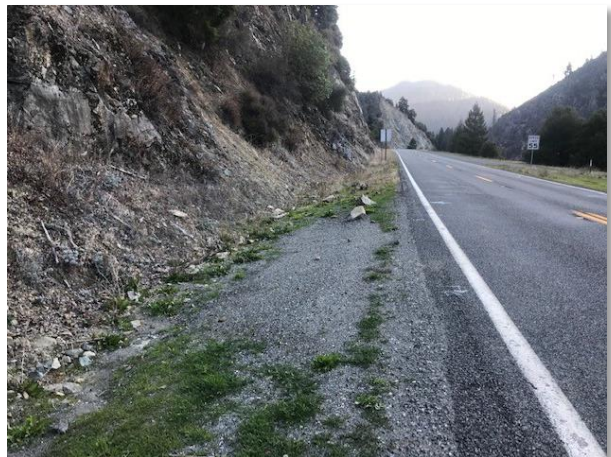
Figure 12. Clean drill and tie-in location with minimal disturbance in Phase 1 (October 31, 2019)
