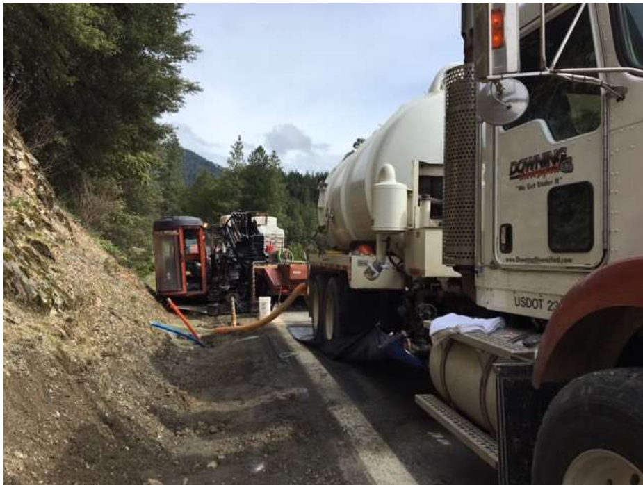
Figure 6 – Drilling south at MP 28.5 – view north, April 3, 2019.
