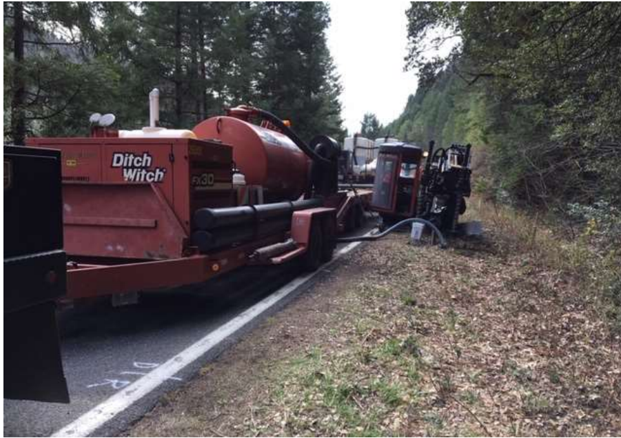
Figure 3 – HDD pulling cable – view south, March 19, 2019.
