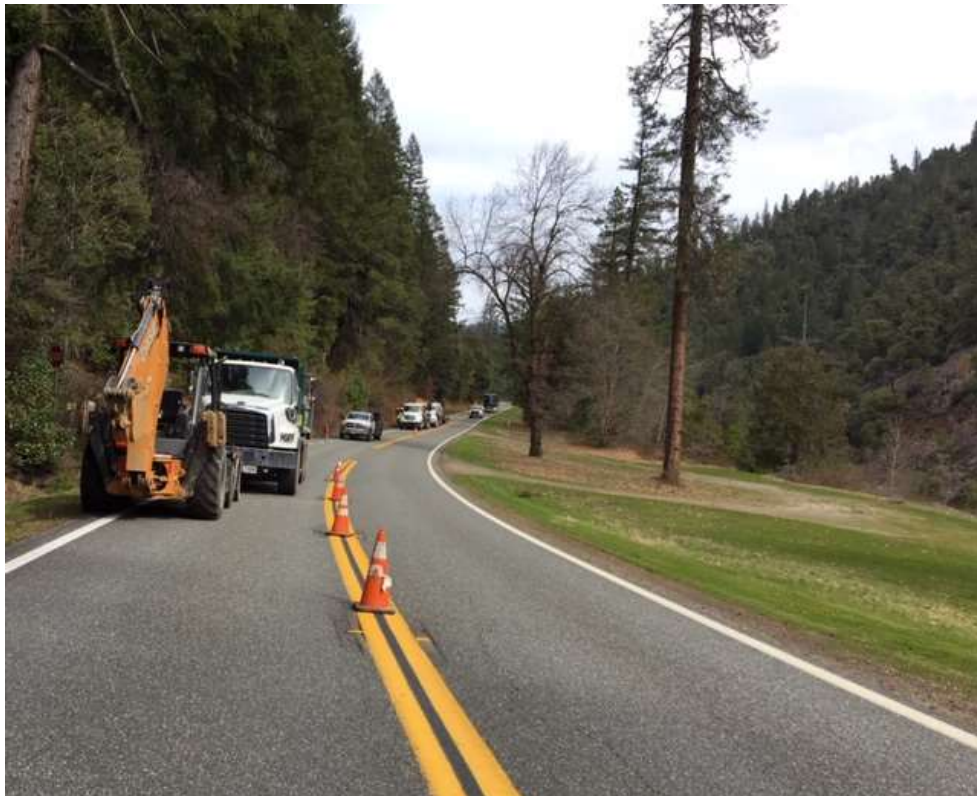
Figure 2 – HDD operations set-up on Hwy 96 – view north, March 19, 2019.
