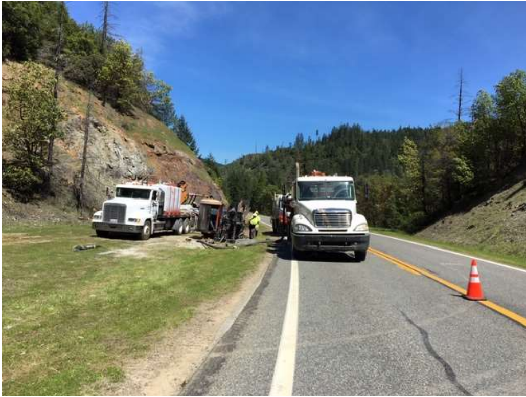
Figure 1 – Crew drilling at MP 26.29 south along Hwy 96 – view north, April 24, 2019.
