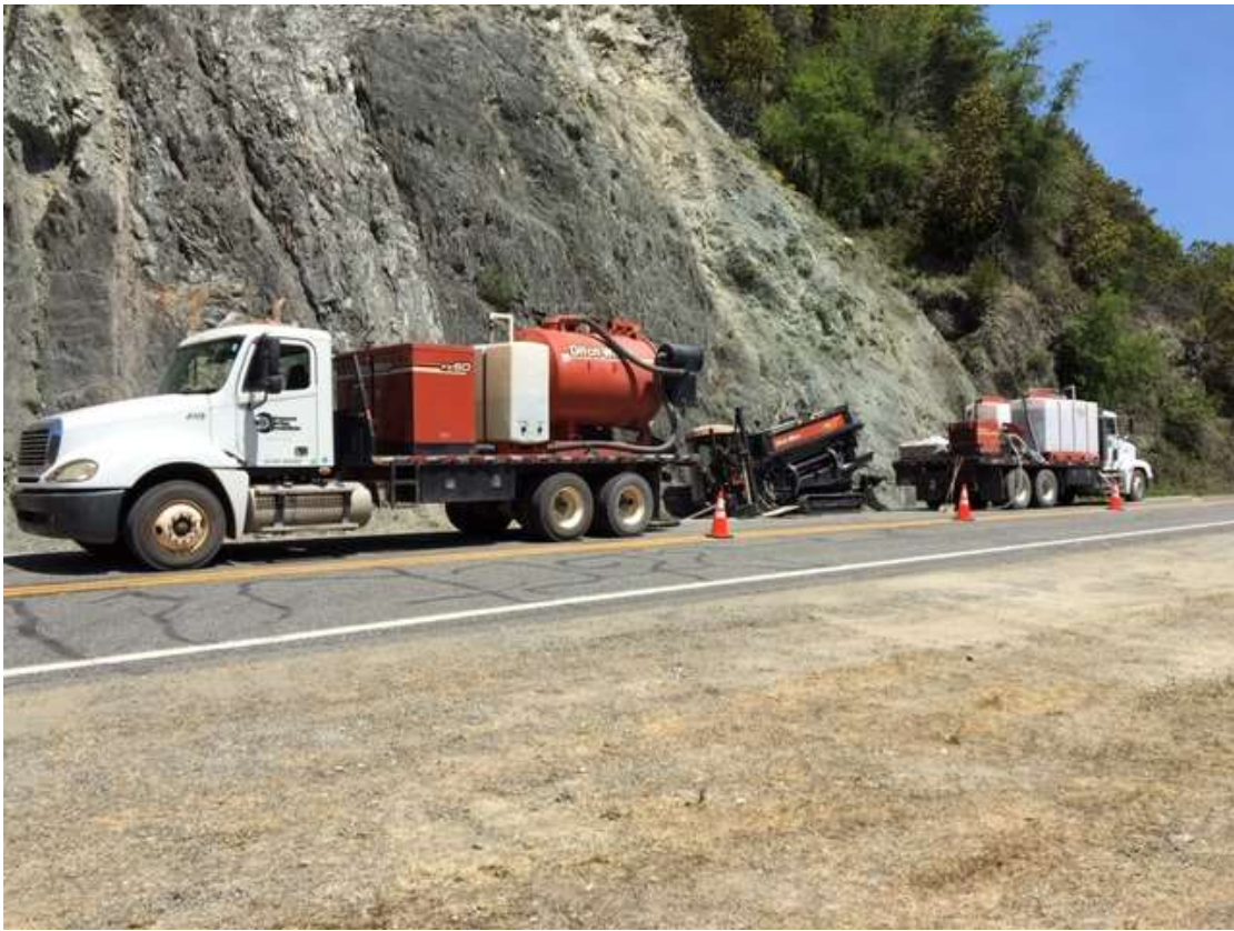
Figure 3 – HDD crew drilling south at MP 25.19 – view northwest, May 9, 2019.
