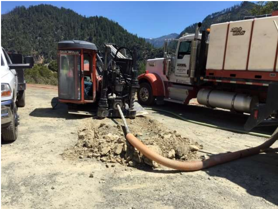
Figure 4 – HDD crew drilling south at MP 25.3 – view northeast, May 9, 2019.
