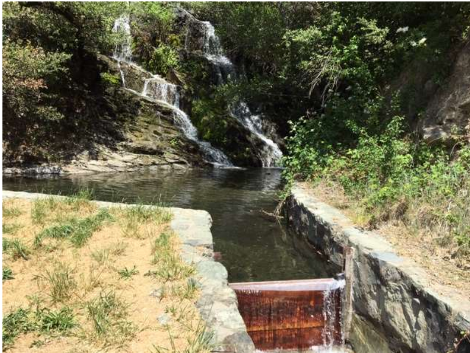
Figure 6 – Wyman Gulch dammed at MP 24.4 – view west, May 9, 2019.
