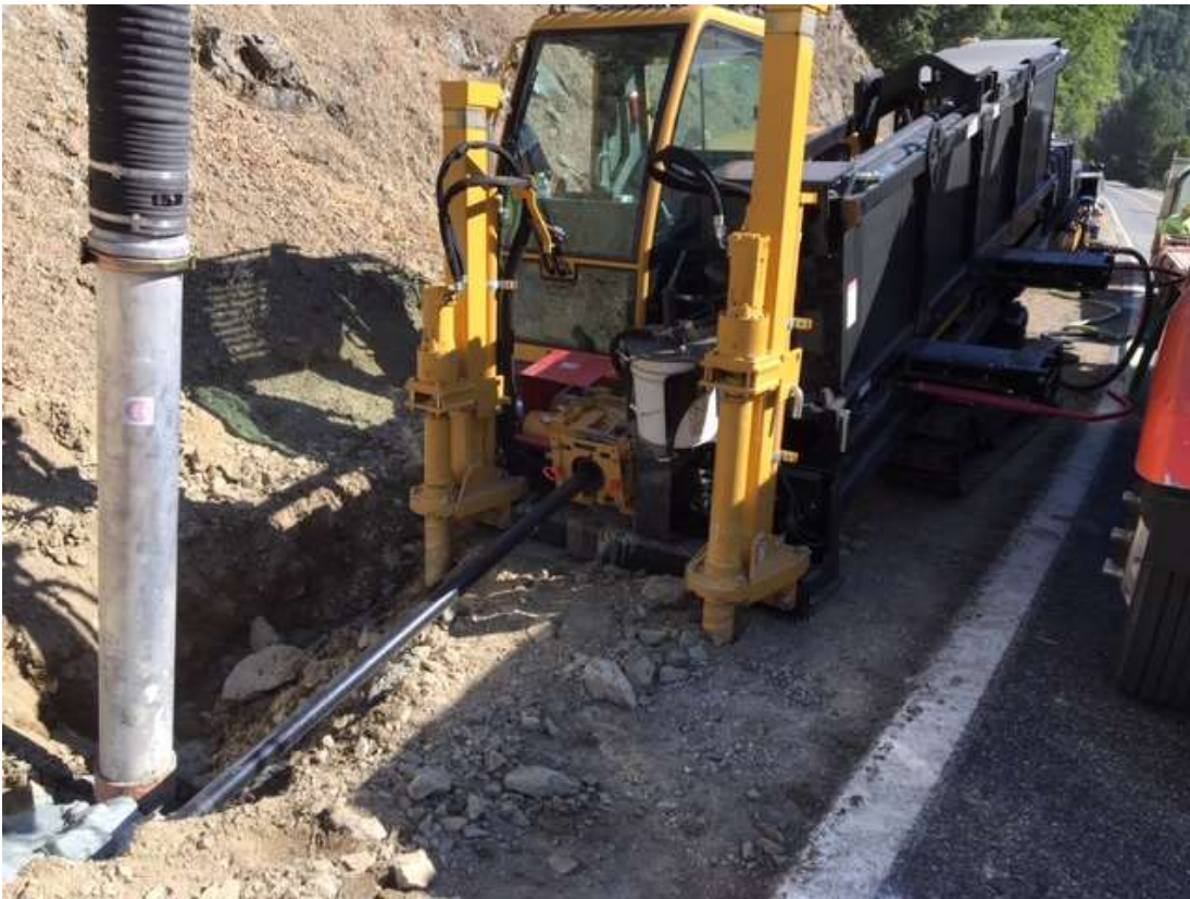
Figure 3 – Crew drilling at MP 23.6 southwest along Hwy 96 – view north, July 10, 2019.
