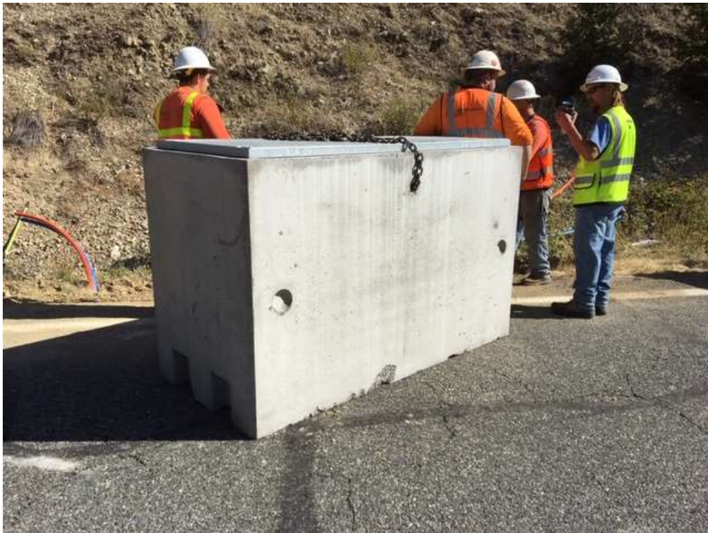
Figure 2 – Crew installing tie-in-box at MP 24.08 – July 10, 2019.
