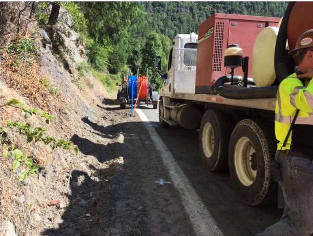
Figure 4 – Crew pulling conduit from MP 23.85 to MP 23.77 – view north, July 10, 2019.
