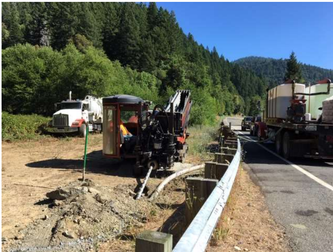
Figure 4 – Crew boring south of Swillup Creek at MP 23.25, view north, July 24, 2019.
