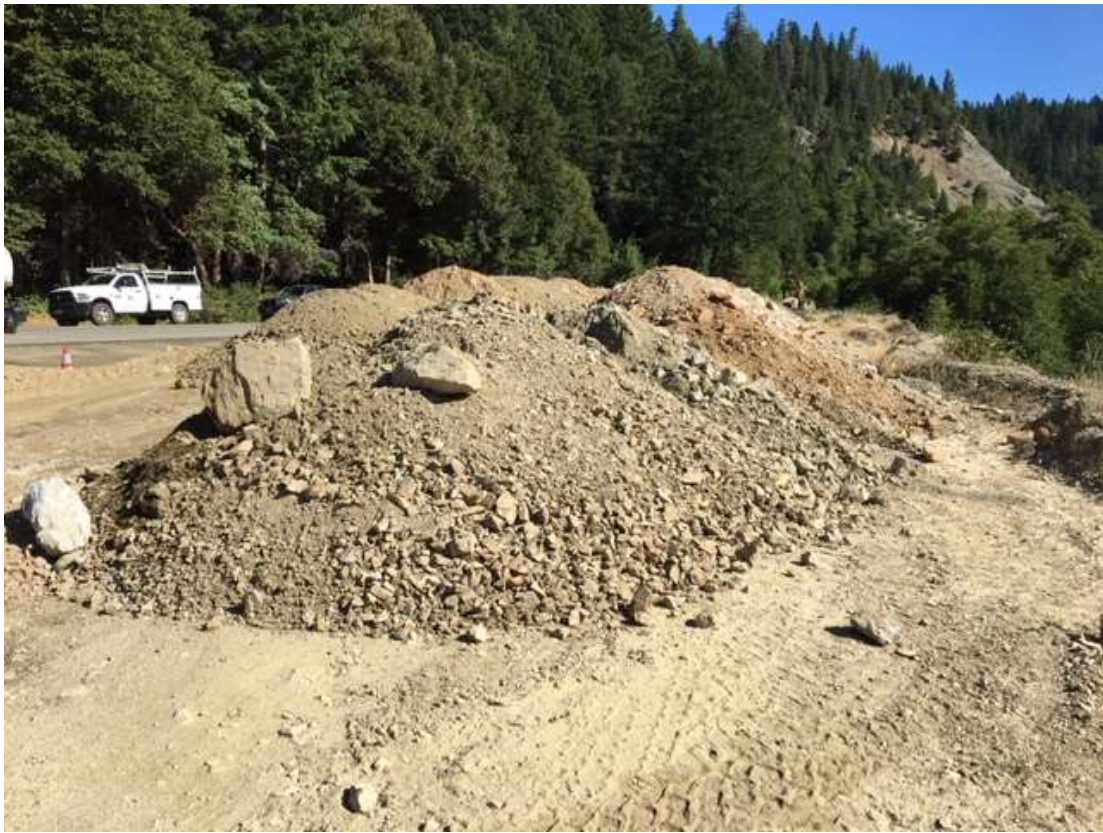
Figure 3 – Temporary storage area of spoils from excavations – July 24, 2019.
