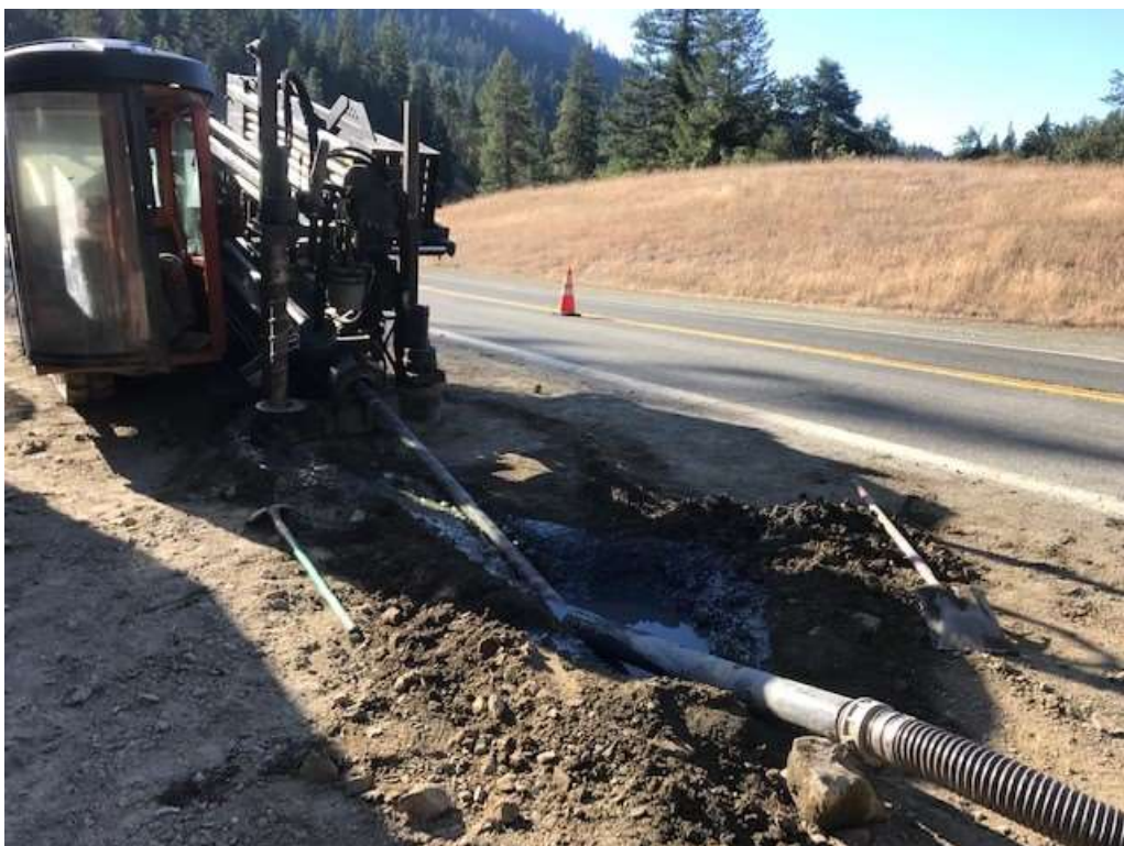
Figure 2 – Third crew drilling north at MP 15.08 – view south, September 11, 2019.
