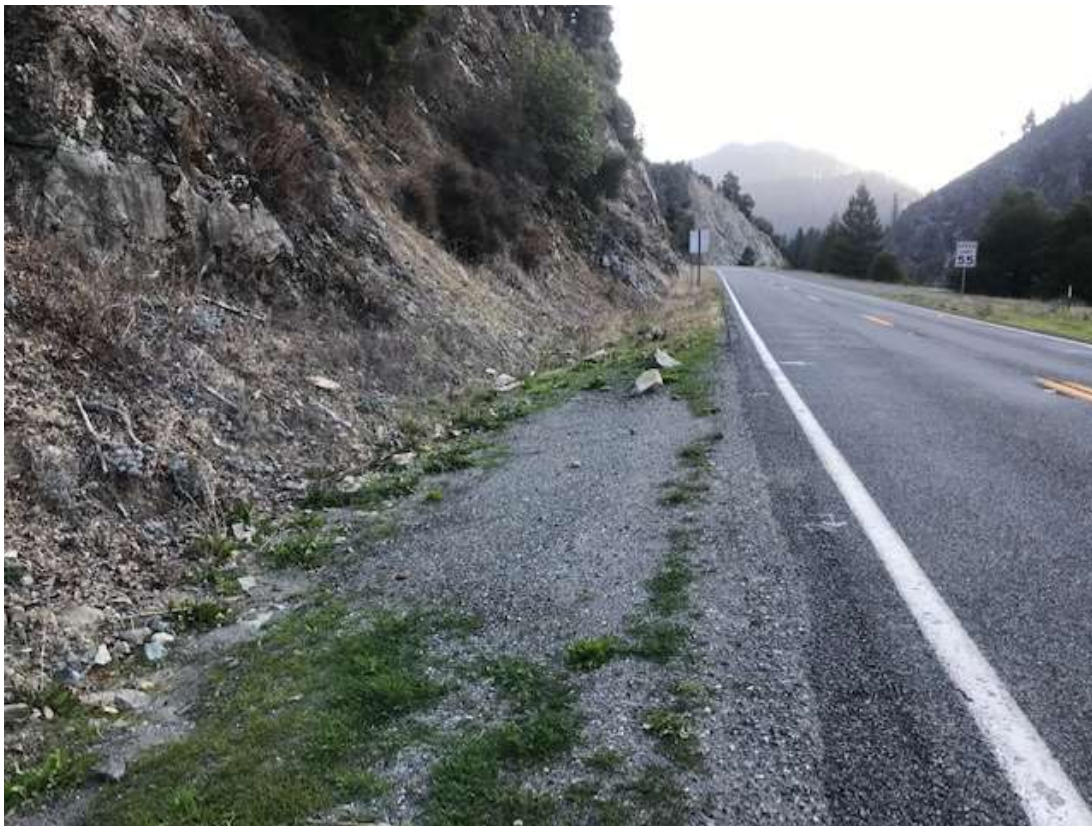
Figure 7 – Clean drill and tie-in location with minimal disturbance in Phase 1, October 31, 2019.
