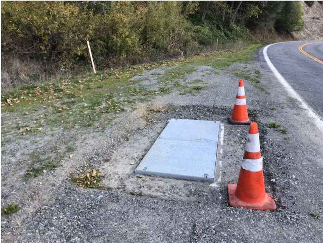
Figure 8 – Tie-in box still needing paving in Phase 2, October 31, 2019.
