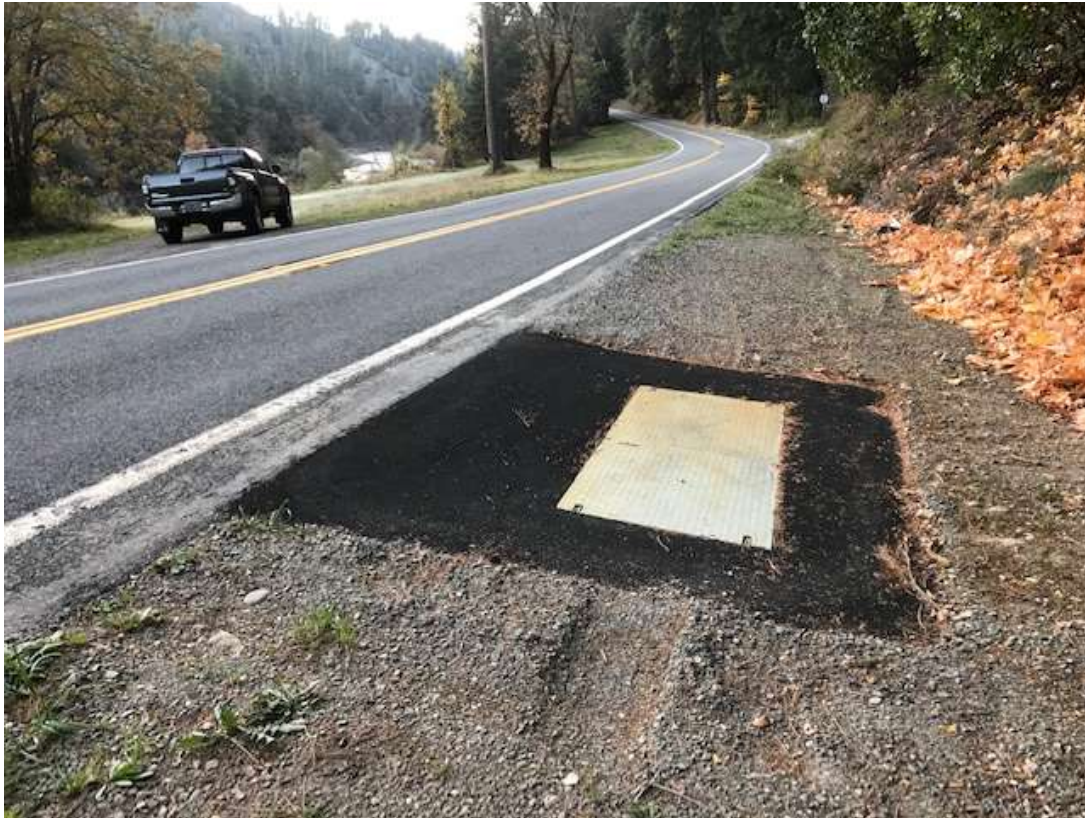
Figure 6 – Clean drill and tie-in location in Phase 1, October 31, 2019
