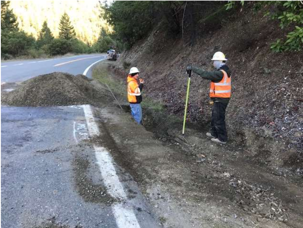
Figure 10 – Crew hand digging tie-in at MP 13.41, October 31, 2019.
