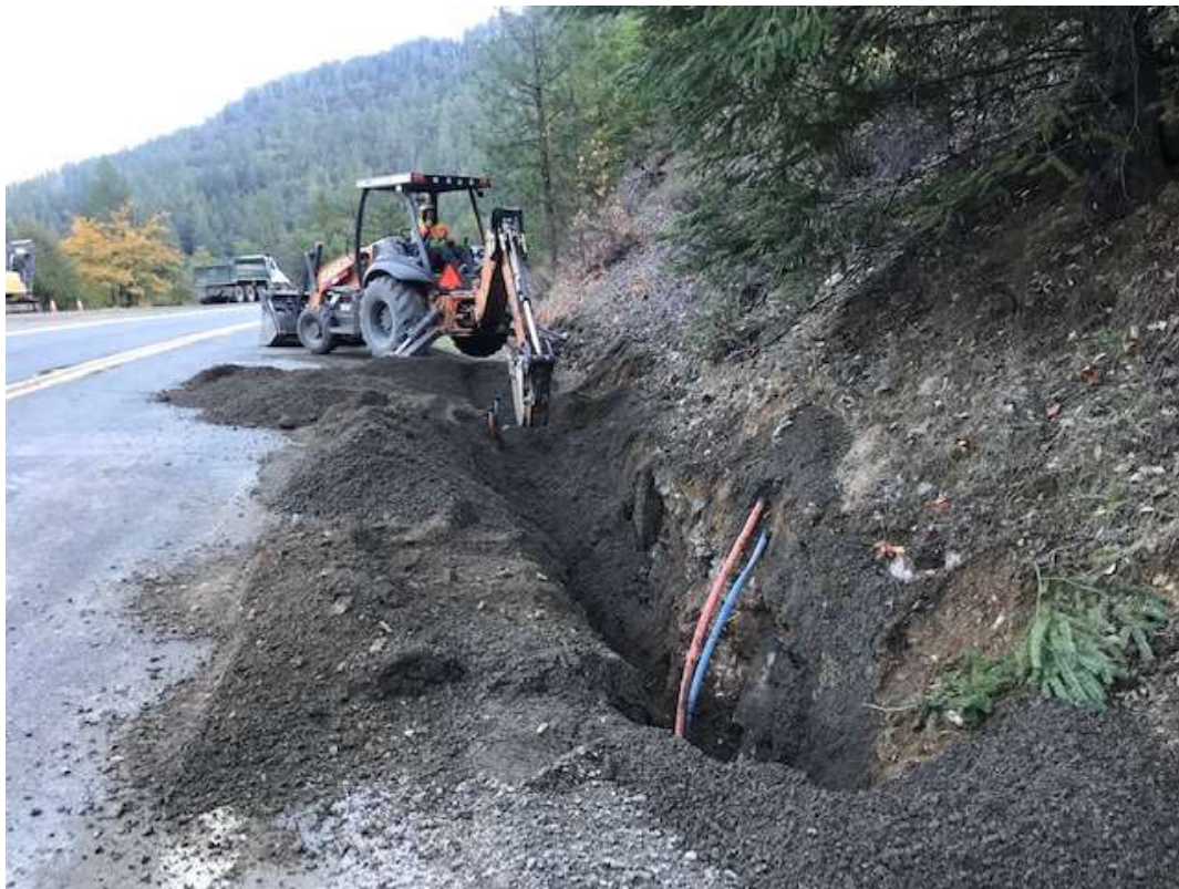
Figure 9 – Crew trenching with a backhoe at MP 13.52, October 31, 2019.
