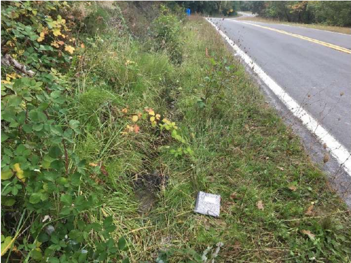
Figure 3 – Cleaned up location within sensitive habitat where nominal frac-out of bore mud occurred at MP 14.15, October 24, 2019.
