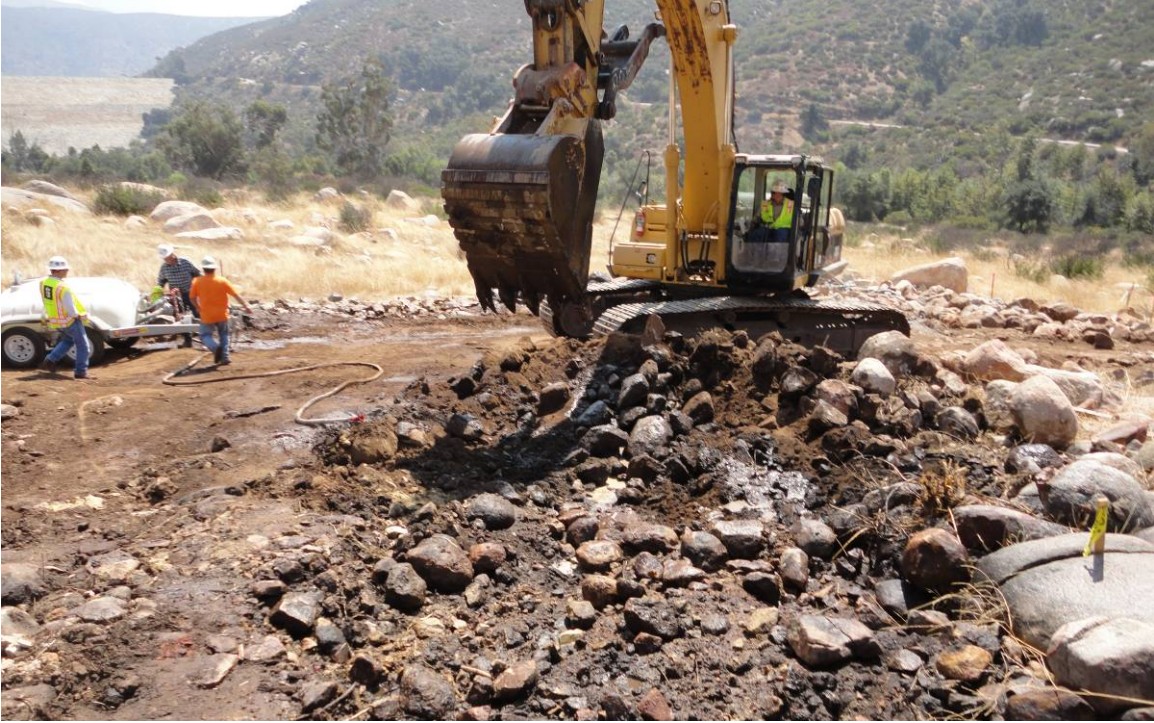
Figure 4. Grading of tower pad for CP70 in unnamed older alluvium; Link 5.
