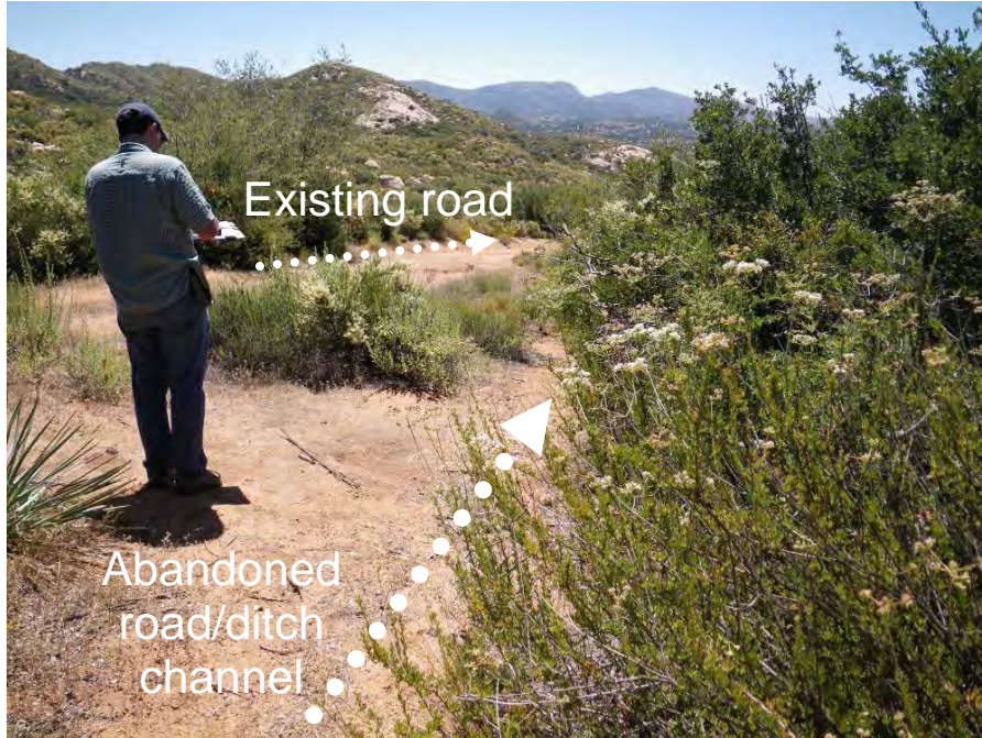
Figure 18. At Site 2-A looking downstream along abandoned road/ditch channel towards its confluence with the existing roadway. At the road, this channel continues along an inboard ditch.
