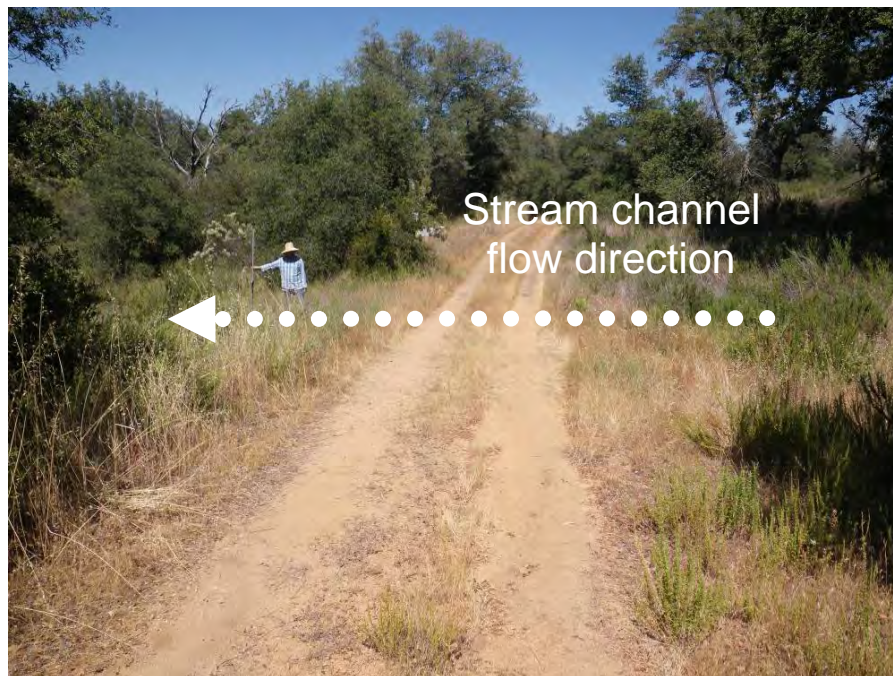
Figure 13. At Site 8 looking east along the existing road at the crossing of the western ephemeral stream (flow is right to left). Note that there is minimal impoundment on the upstream side of the crossing (right side of photo) and minimal channel drop on the downstream side (left side of image).
