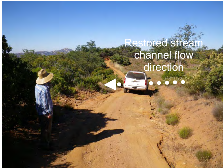
Figure 27. View of same road crossing shown in Figure 26 at Site 11. Road cut areas will be filled to restore the natural topography surrounding the stream channel valley.
