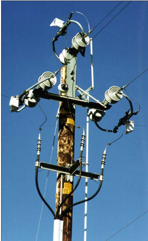
Figure 3-12 600 Amp KPF Air Switch, Triangular Construction (closed position)
