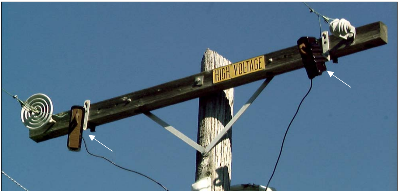
Figure 2-7 Arm Mounted Enclosed Cutout with Universal Fuses
