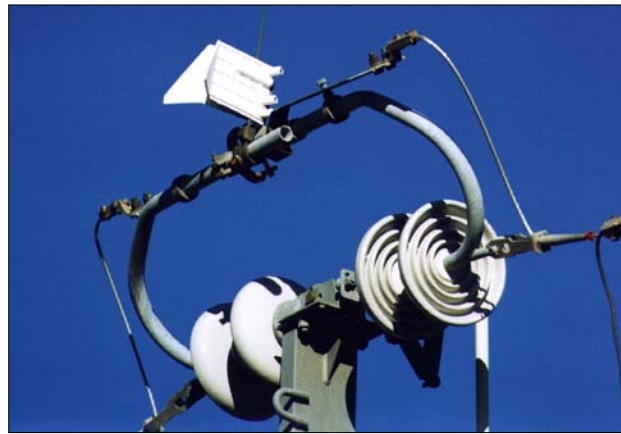
Figure 3-12 600 Amp KPF Air Switch, Triangular Construction (closed position)
