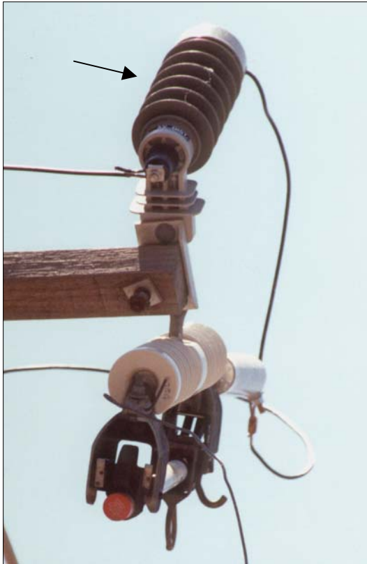
Figure 2-20 Non-Porcelain Lightning Arrester
