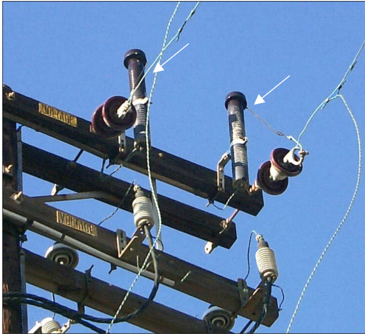
Figure 2-24 Lightning Arrester
