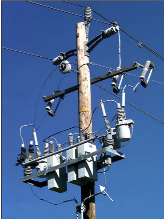
Figure 3-29 Capacitor Bank
