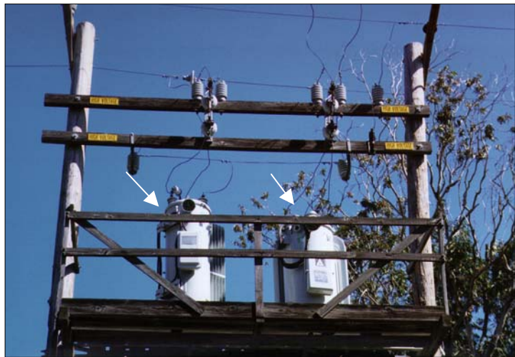
Figure 3-28 Voltage Regulator
