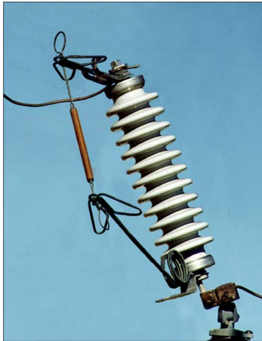
Figure 2-5 Bushing Mounted Cutout with Open Link Fuses
