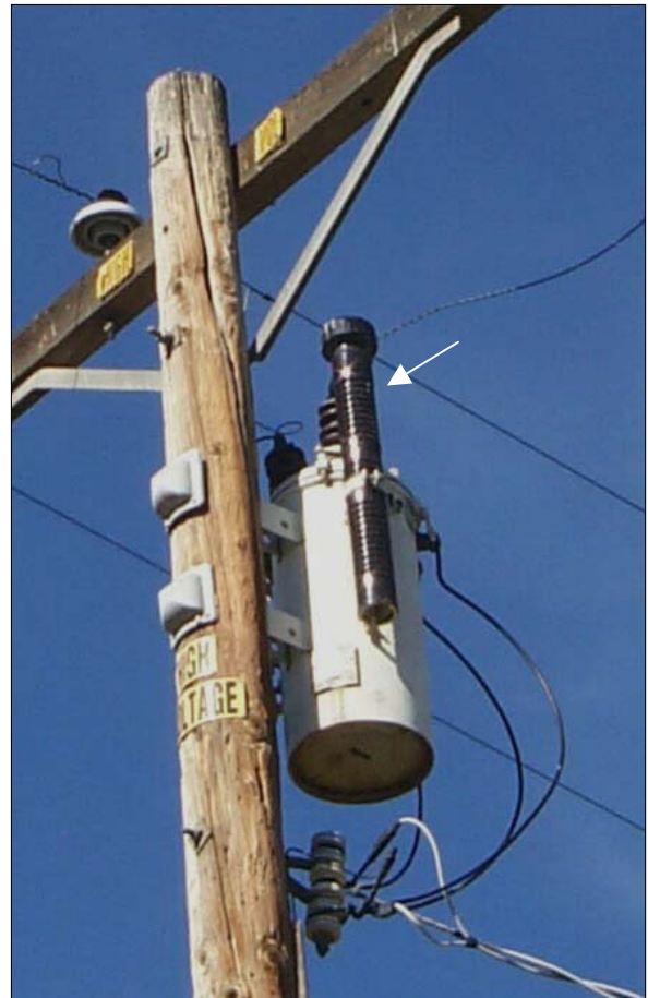
Figure 2-25 Lightning Arrester
