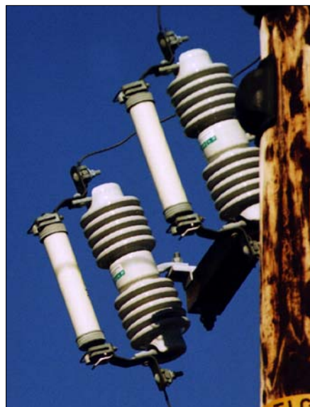
Figure 3-1 Arm Mounted Cutout with Non-Expulsion Fuse
