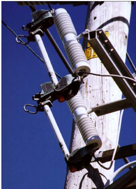
Figure 3-8 Arm Mounted Cutout with SMU-20 Fuses
