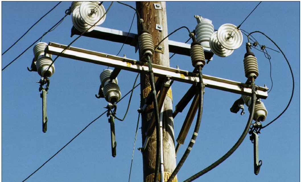
Figure 2-9 Arm Mounted Cutout with Solid Blade Disconnect (open position)
