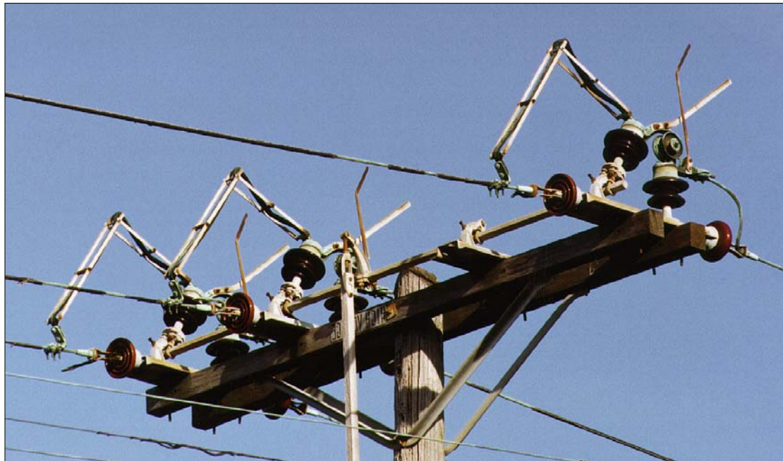
Figure 2-31 Grasshopper Air Switch (closed position)
