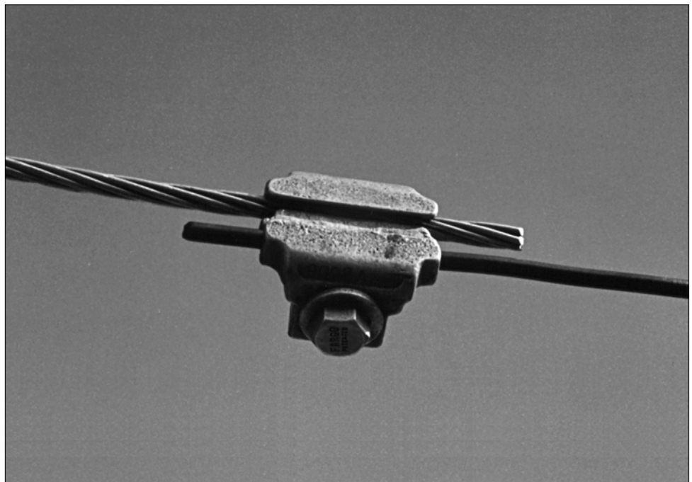
Figure 2-30 LM Connector
