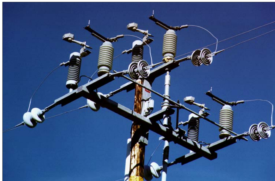
Figure 3-20 S&C Omni-Ruptor Switch, Triangular Construction (open position)
