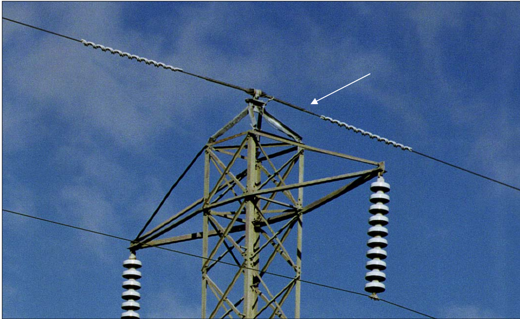
Figure 4-27 Tangent Transmission Tower with Static Line
