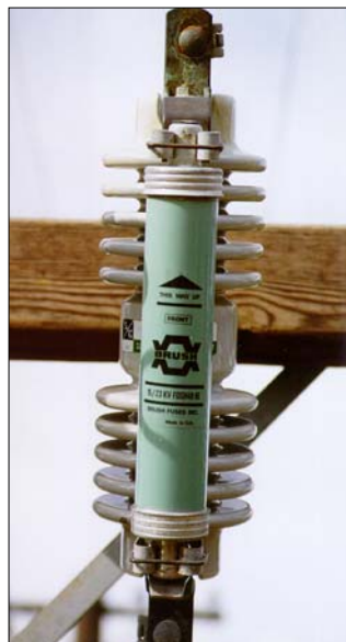
Figure 3-2 Arm Mounted Cutout with Non-Expulsion Fuse
