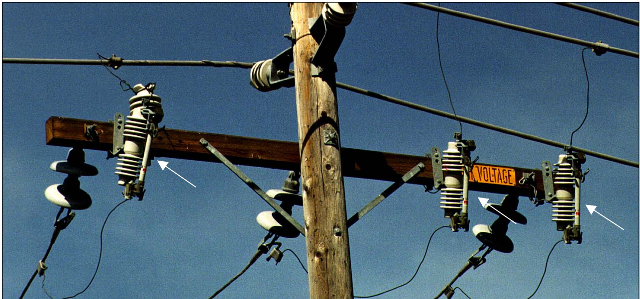
Figure 2-3 Arm Mounted Cutout with Universal Fuses
