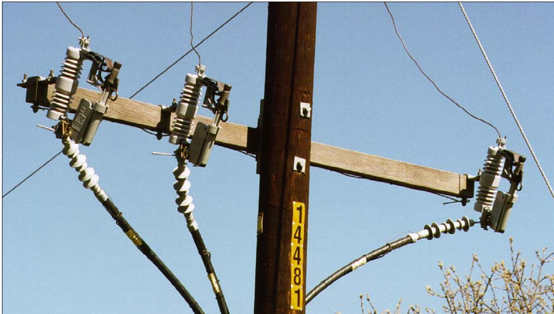
Figure 3-11 Arm Mounted Cutout with S&C Fault Tamer Fuse
