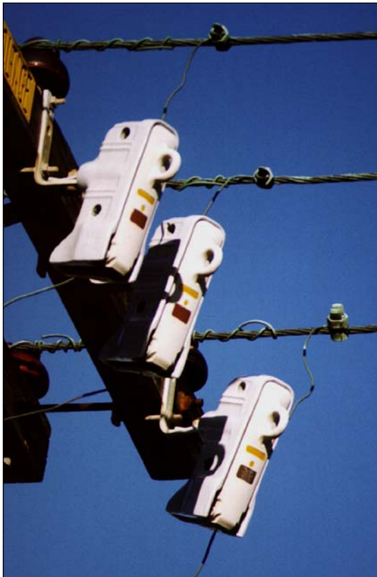
Figure 2-6 Enclosed Cutouts
