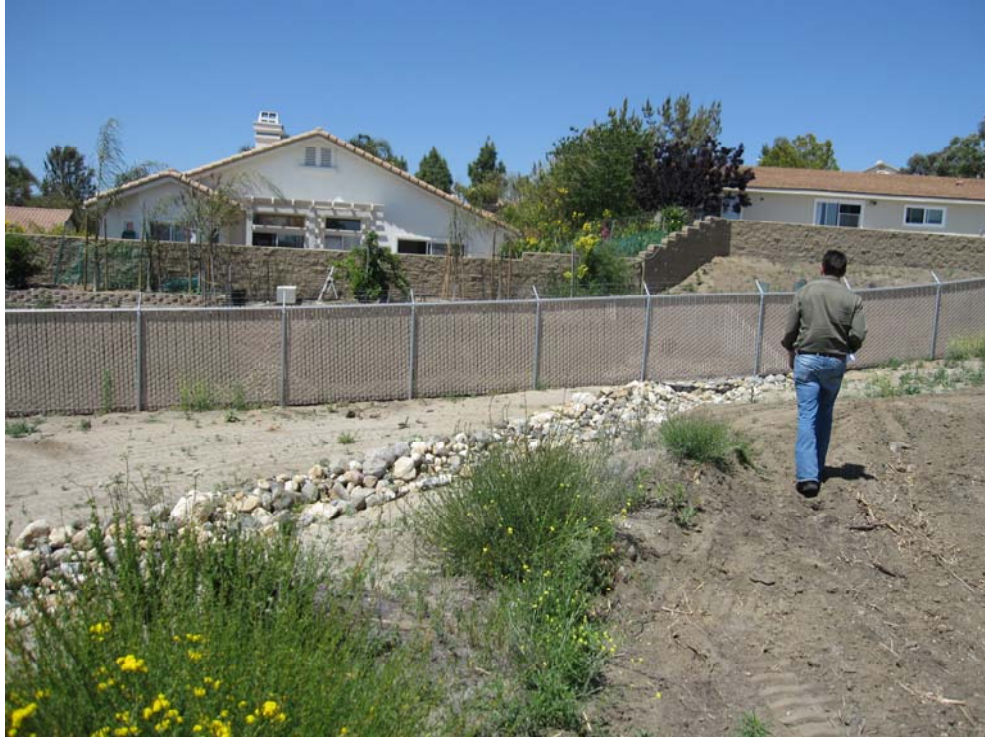
Offsite run-on north side of Storage Yard
