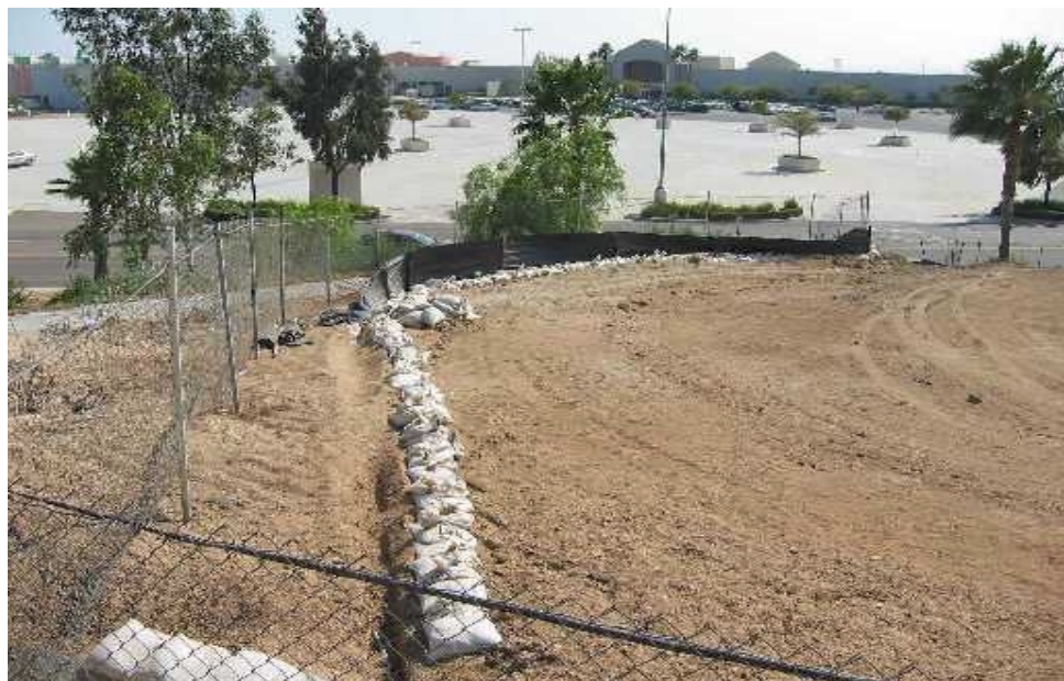
Gravel bags used as perimeter control.
