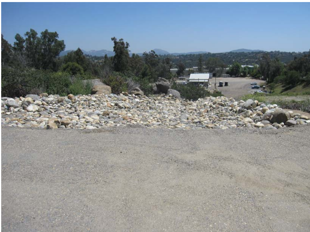
Rock swale on southwest side of Storage Yard
