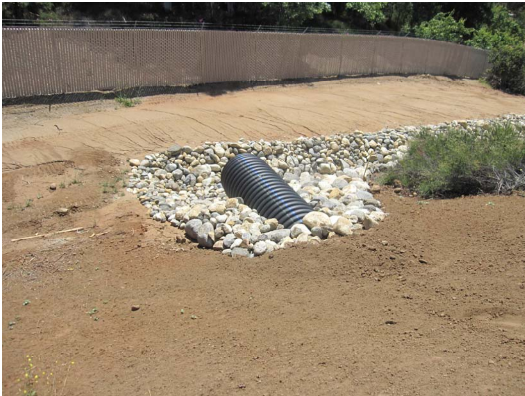
Rock swale south side of Storage Yard
