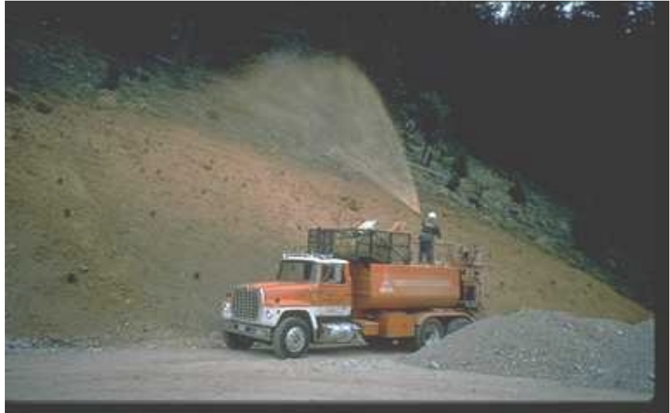
Applying hydraulic mulch.
