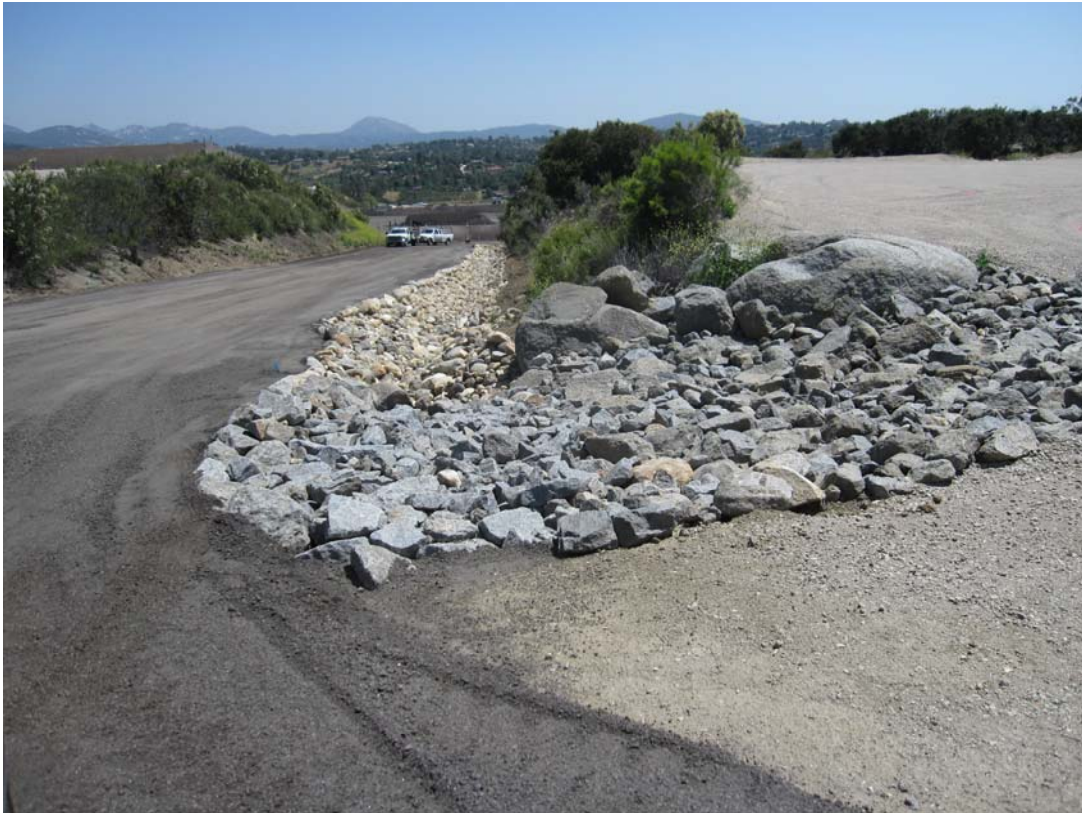
Rock swale on east side of access road to Storage Yard
