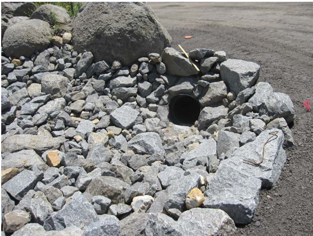
Rock swale and pipe inlet on west side of Storage Yard
