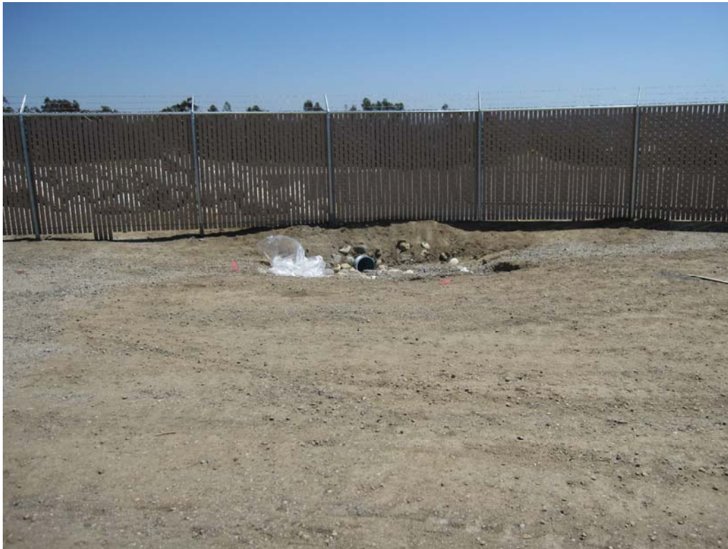
Pipe inlet southwest side of Storage Yard
