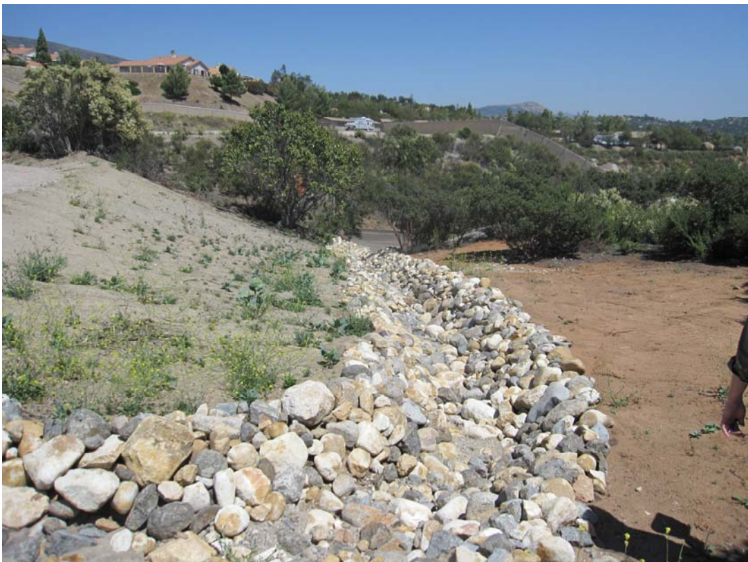
Rock swale on south side of Storage Yard
