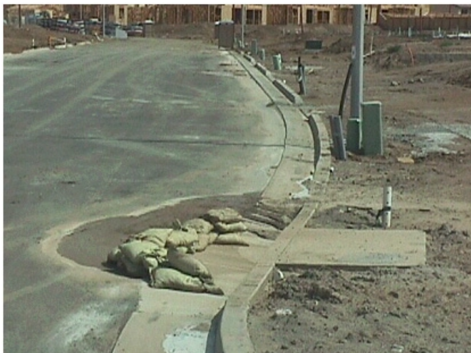
Gravel bag inlet protection.
