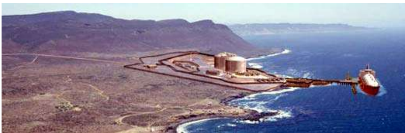
Sempra’s Energia Costa Azul LNG terminal storage tanks 14 miles north of Ensenada Mexico.
