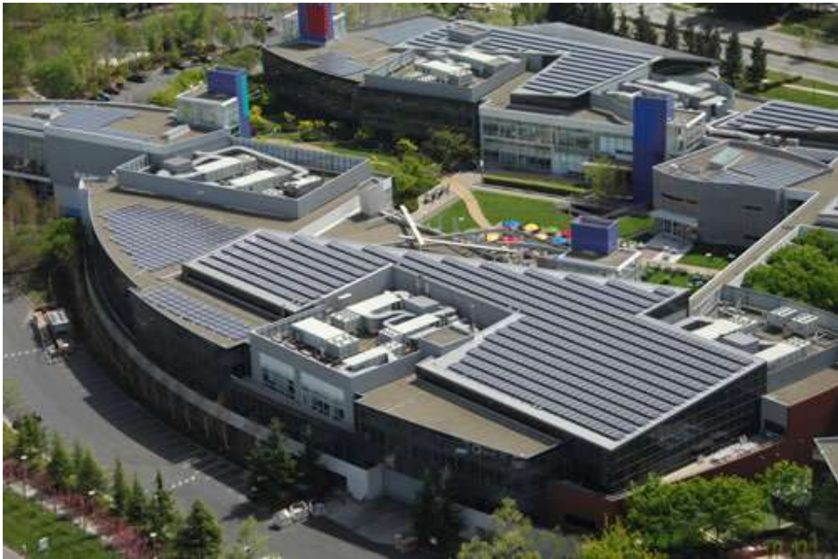
1.6 megawatts of solar generation on the roof of Google's offices
