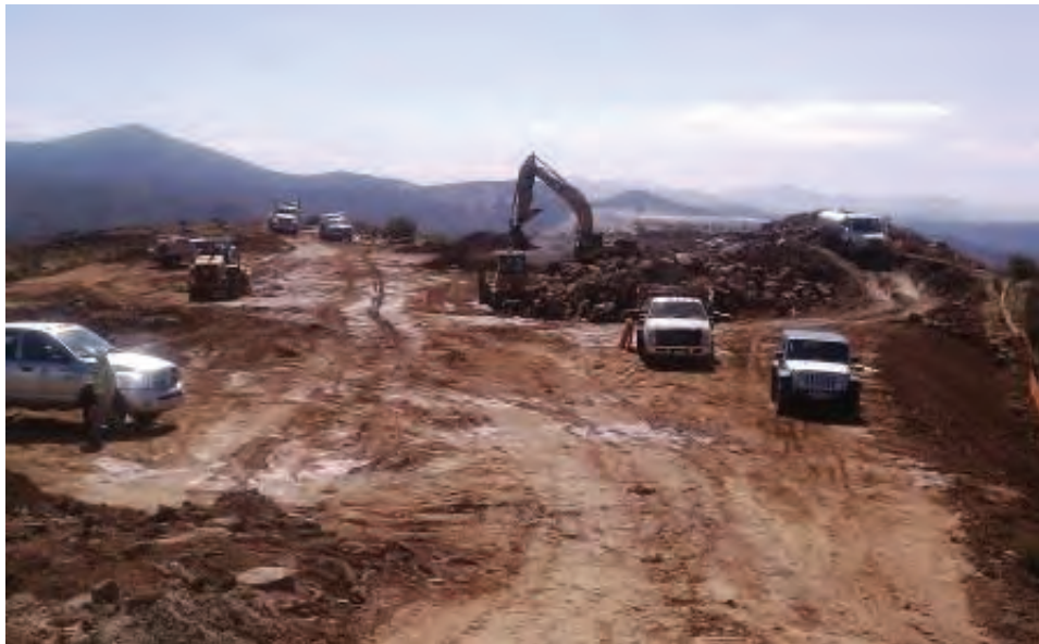
Figure 12: Boulder busting at Barrett Construction Yard. (Link 2)
