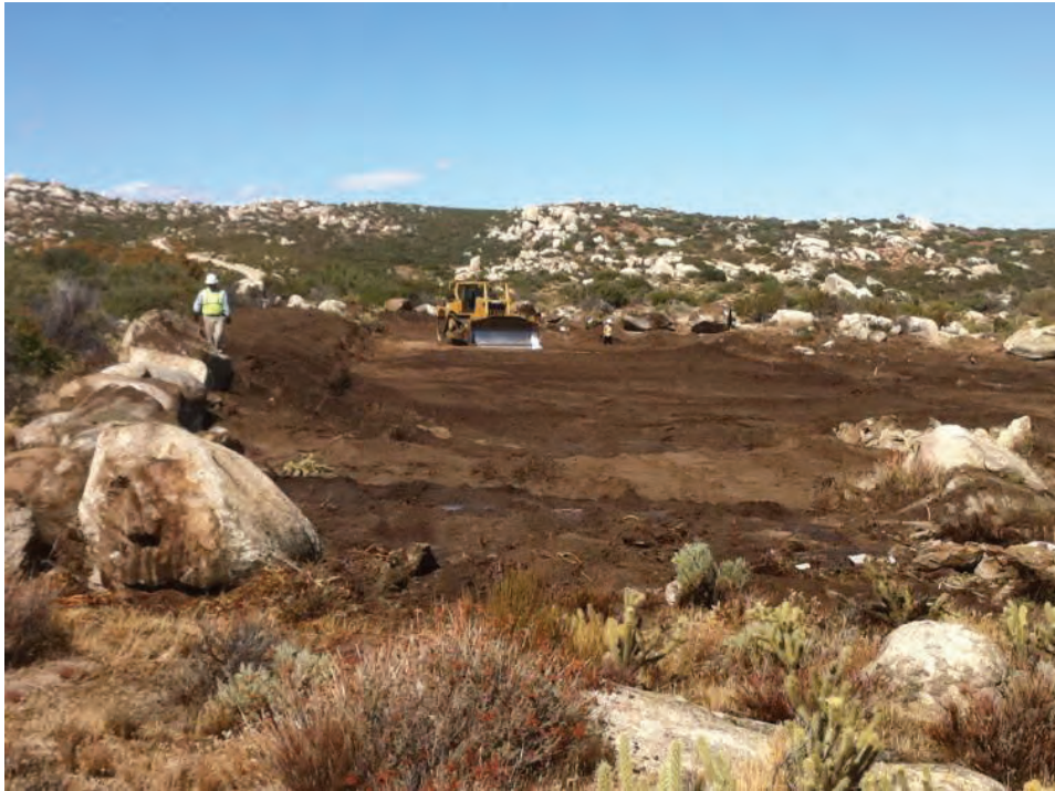
Figure 1: Grading EP187-2 pull site. (Link 1)
