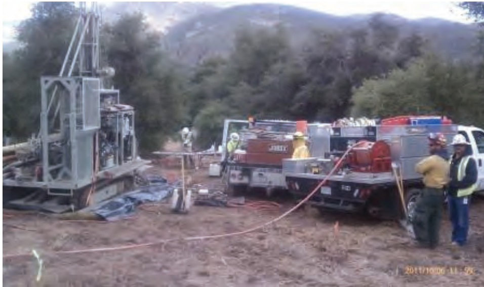
Figure 4: Soil boring at EP141. (Link 2)
