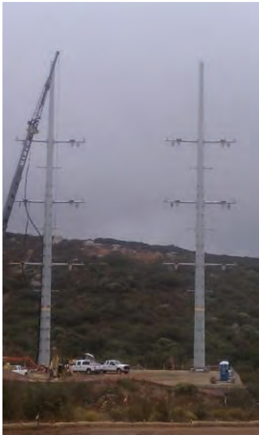
Figure 5: Cable pulling at riser poles CP95-1 and CP96-1. (Link 4)
