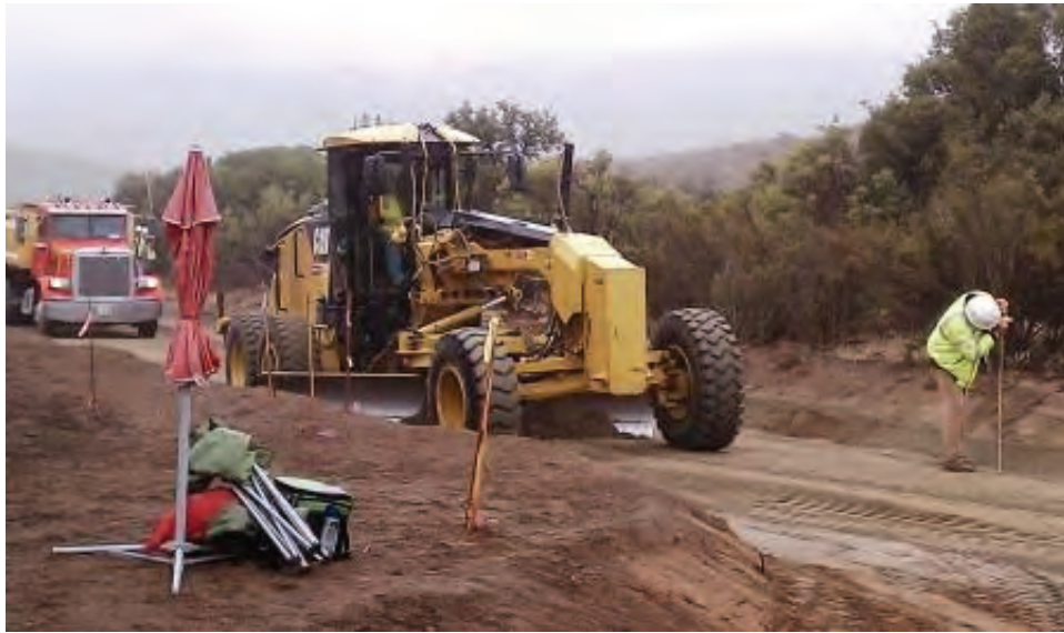
Figure 3: Laying down road base on La Posta Road. (Link 2)
