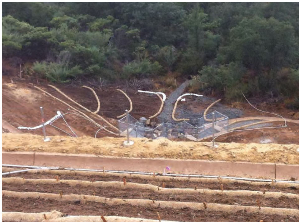
Figure 8: BMP installation at the northern dissipater. (Link 3)
