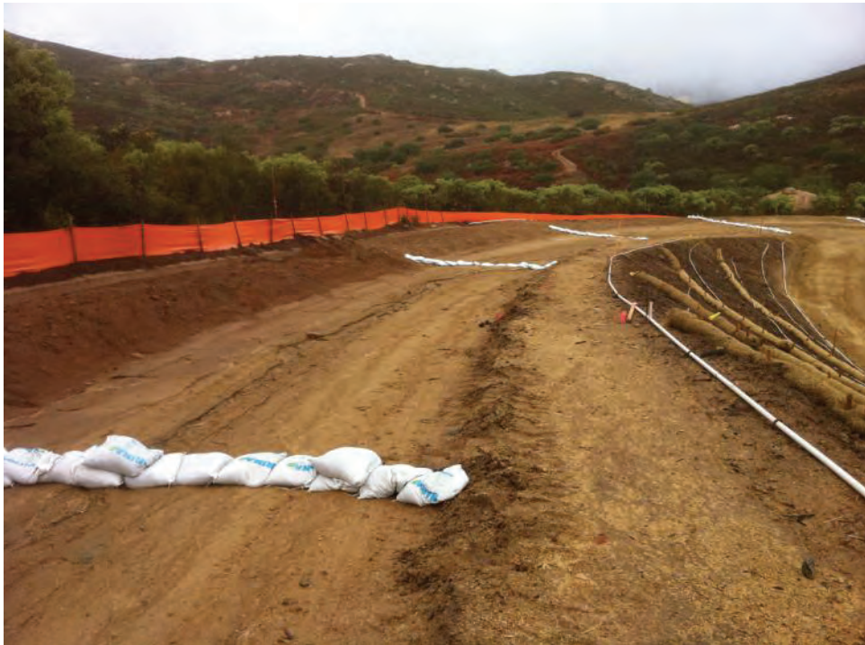
Figure 9: Gravel bags placed at unfinished access road, post-rain event. (Link 3)
