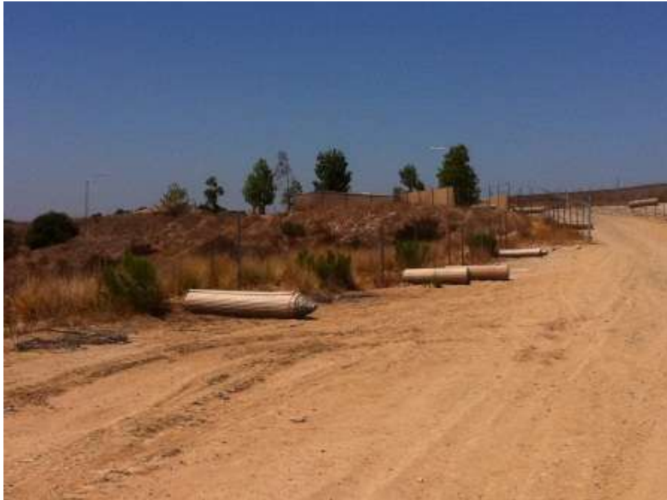
Figure 2: Fence removal at Sycamore Yard. (Link 5)
