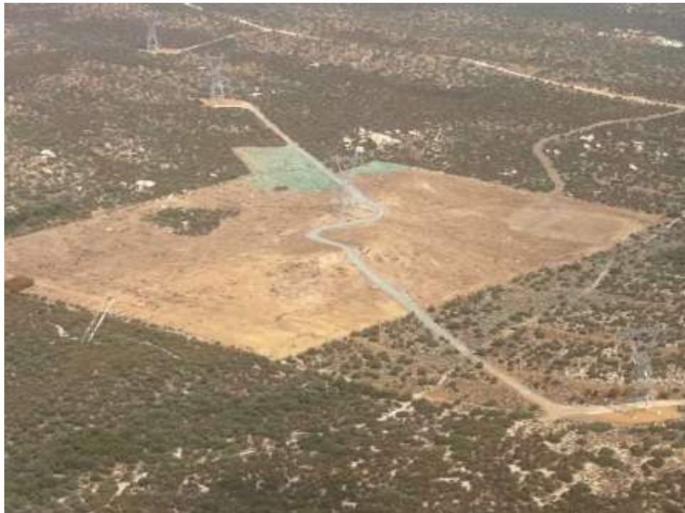
Figure 4: Hydromulching at McCain Valley Yard. (Link 1)
