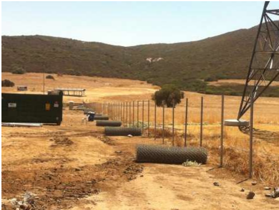
Figure 3: Fence removal at SWAT Yard. (Link 2)
