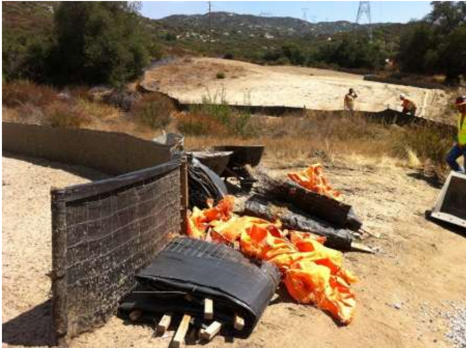
Figure 1: Clean up occurred at EP78/EP79 pull site. (Link 1)
