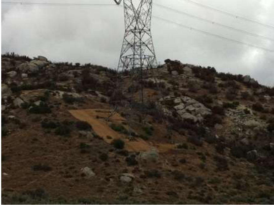
Figure 1: Coco blanket installation at EP117-2. ( Link 1 )
