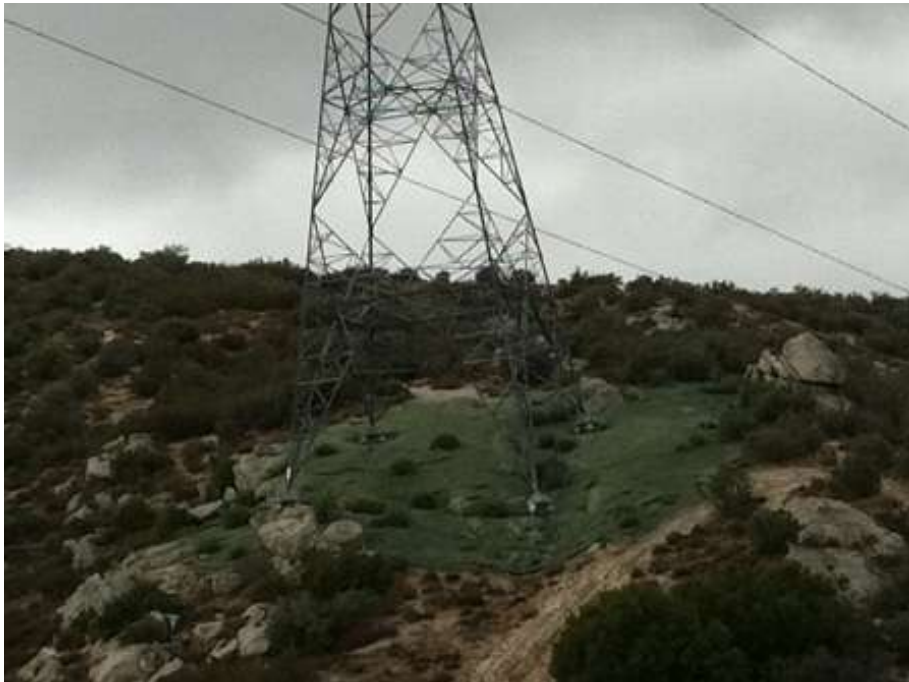
Figure 2: Hydromulching at EP115-1. ( Link 2 )
