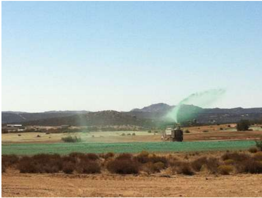
Figure 3: Hydromulching at Rough Acres Yard. (Link 1)
