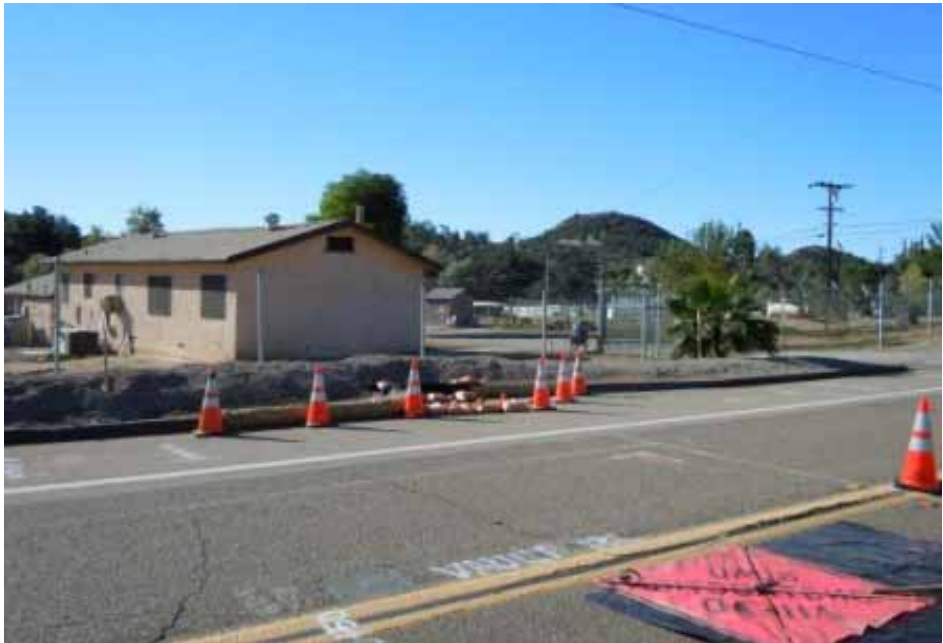
Figure 2: BMPs installed along Alpine Boulevard during potholing activities.
