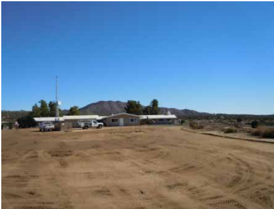
Figure 4: Class II base installed at Rough Acres Construction Yard.
