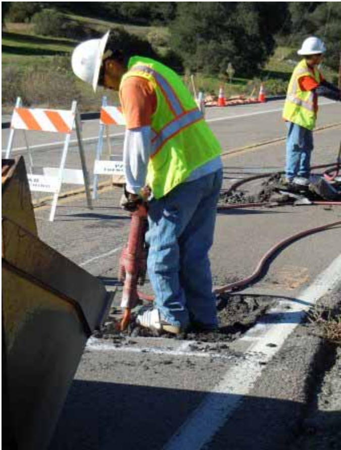
Figure 1: Potholing along Alpine Boulevard.
