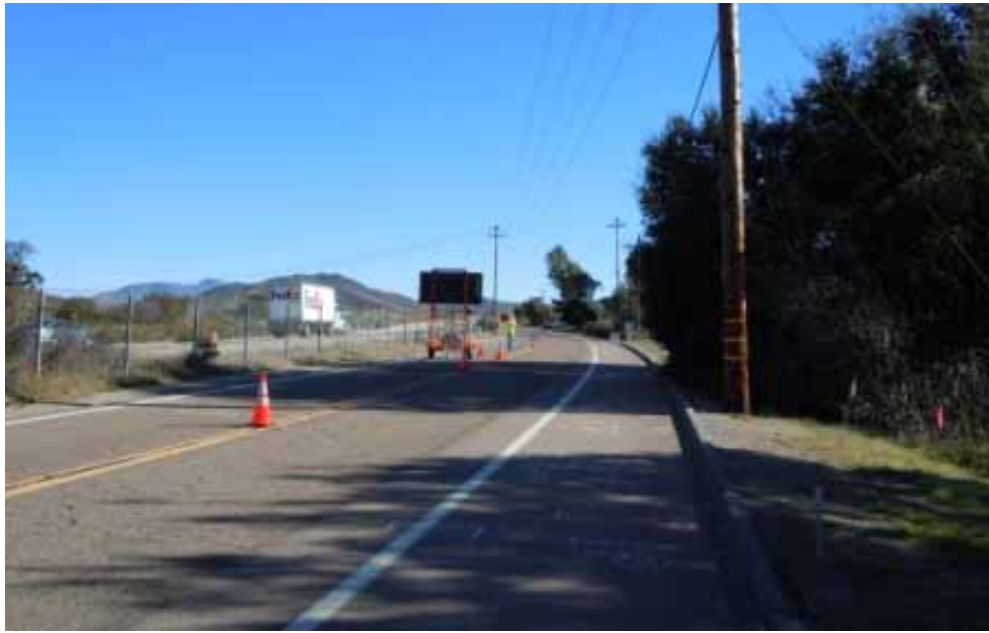
Figure 3: Traffic Control setup during potholing operations on Alpine Boulevard.
