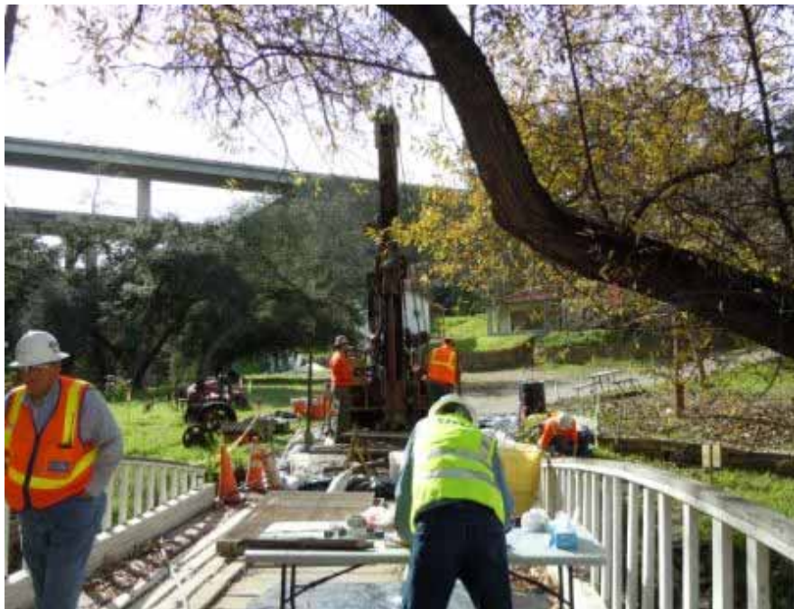
Figure 2: Geotechnical drilling at the Bauer Property, Link 4.
