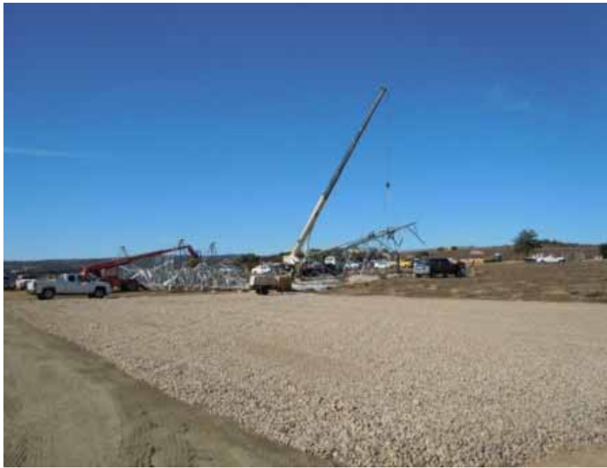
Figure 3: Steel assembly at the Rough Acres Yard.
