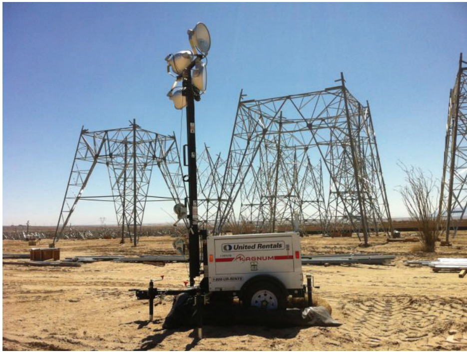
Figure 5: Secondary containment around Light Pots at S2 Construction Yard, Link 1.
