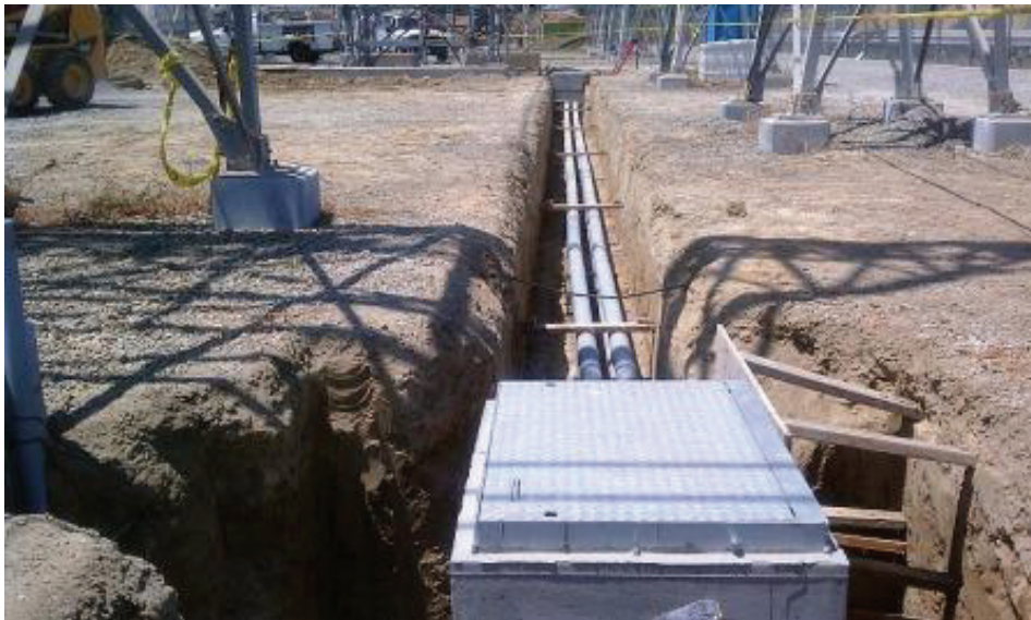
Figure 4: Trenching and conduit installed at the Encina Substation.
