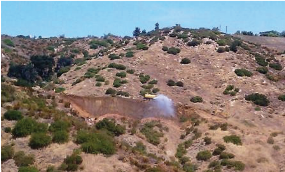
Figure 1: Dust control and grading operations on the Slay Property. (Link 4)
