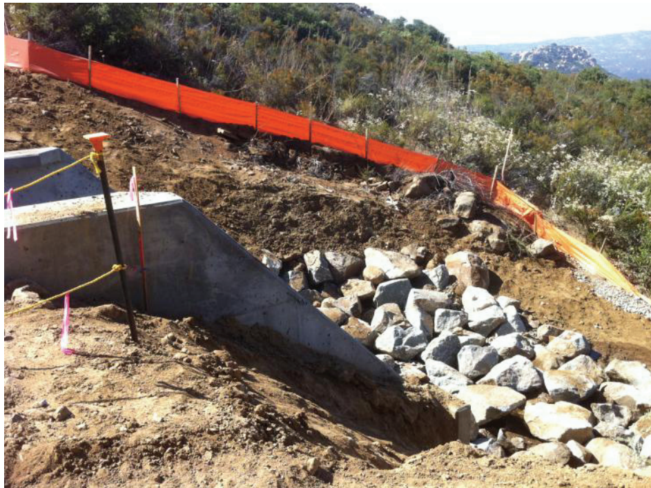
Figure 3: Rip rap installation at Suncrest Substation, Link 3.
