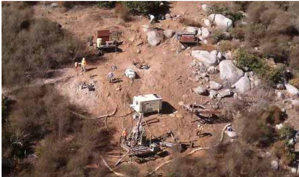
Figure 4: Aerial view of micropile operation at CP72-2. (Link 5)
