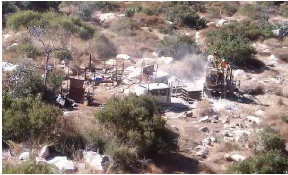
Figure 5: Aerial view of micropile operation at CP66-2. (Link 5)
