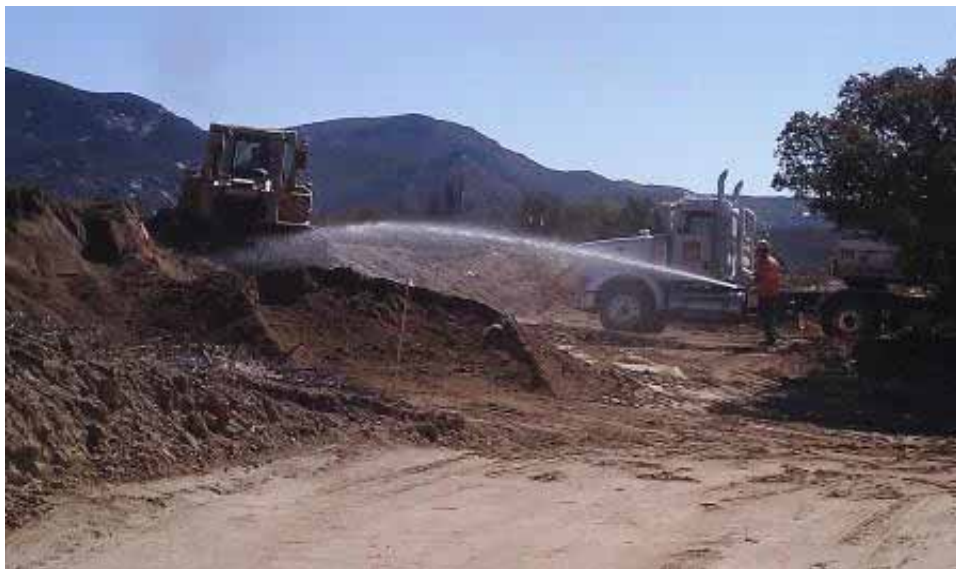
Figure 10: Grading on USFS land at Thing Valley Construction Yard. (Link 2)
