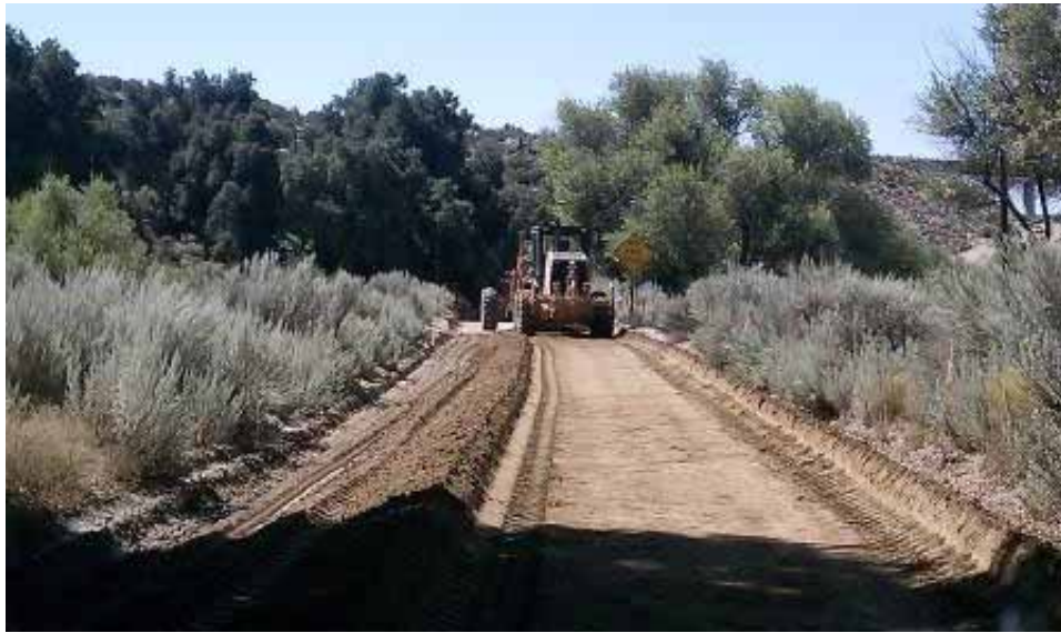
Figure 3: Grading of La Posta Road on USFS land. (Link 2)
