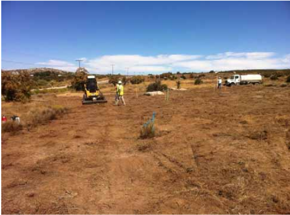
Figure 1: Vegetation clearing at EP207. ( Link 1 )
