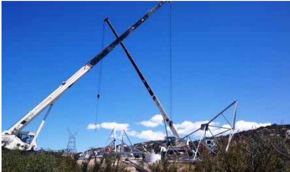
Figure 2: Tower assembly at EP91. ( Link 2 )
