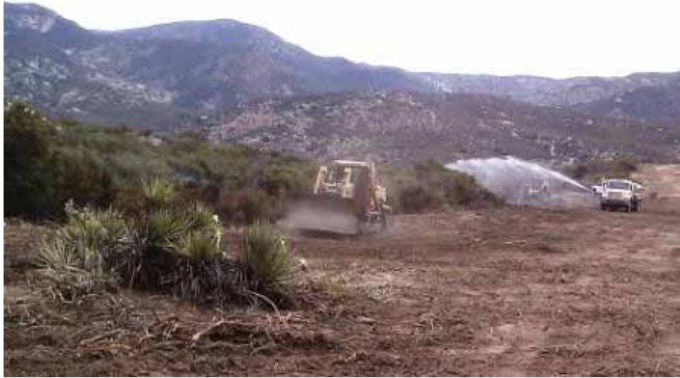
Figure 9: Vegetation clearing on USFS land at Thing Valley Construction Yard. (Link 2)
